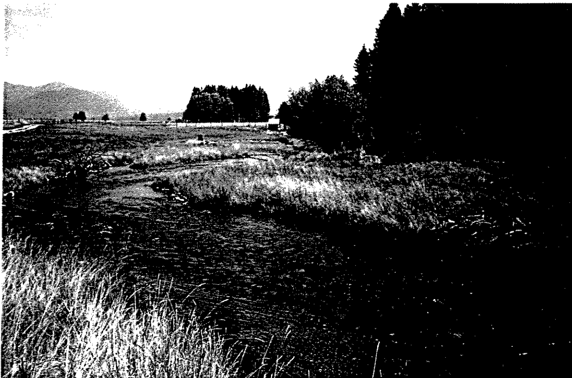
Photo 3. Stream Channel Rehabilitation. The channel of Rock Creek, a spring creek that enters the North Fork of the Blackfoot River, was rebuilt by removing sediment from pools, using excavated material to build point bars and to create a narrower meandering stream. Flow in the narrowed stream channel has greater energy to transport sediment and cleanse spawning gravels. Grass and other vegetation have become established on the streambanks. This photo was taken one year after treatment.
