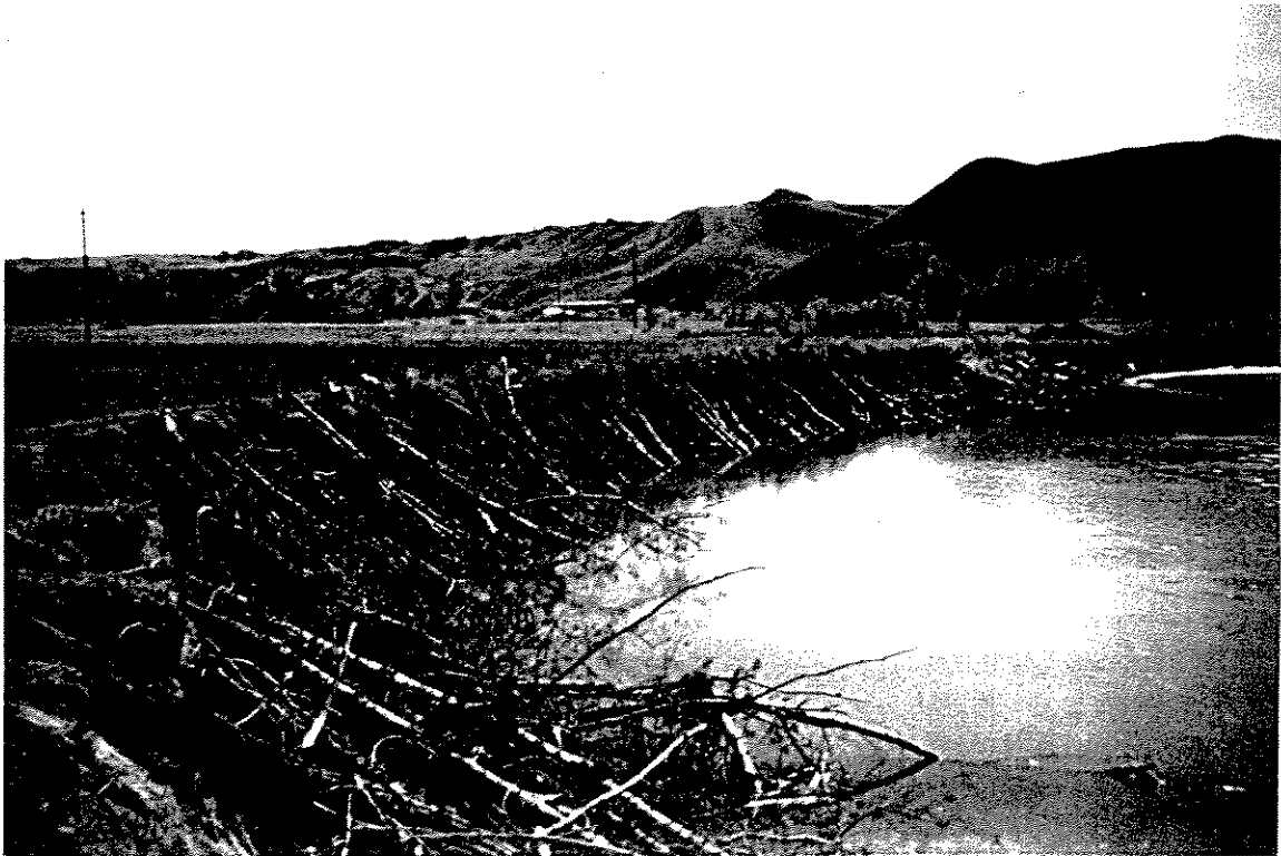
Photo 6. Bank Stabilization. Approximately 1,300 feet of the Marias River was treated with cottonwood logs to stabilize the river bank and prevent erosion of riparian areas and farmland. Small shrubs and other vegetation growing between the cabled down logs will add additional stability to the bank.
