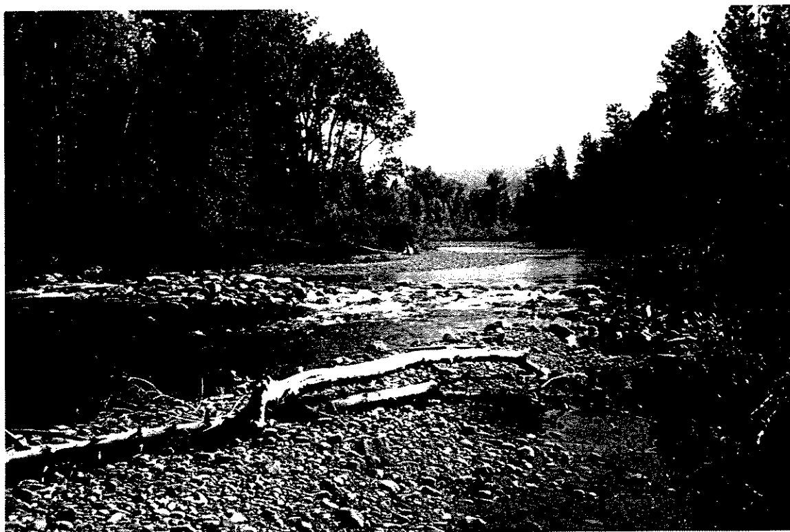
Photo 2. Channel Stabilization and Irrigation Diversion. This rock drop structure on the Big Blackfoot River stabilized the channel as well as providing a permanent rock irrigation diversion structure, thereby eliminating the need for annual maintenance work in the channel. The headgate is off the photo.
