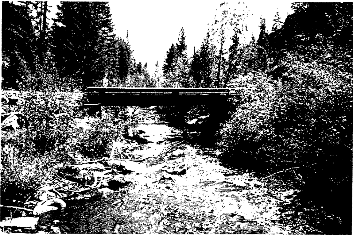
Photo 5. Fish Passage. Fill and culverts on Belmont Creek, a tributary to the Big Blackfoot River, were removed and replaced with a bridge that allowed spawning fish to access upstream reaches.
