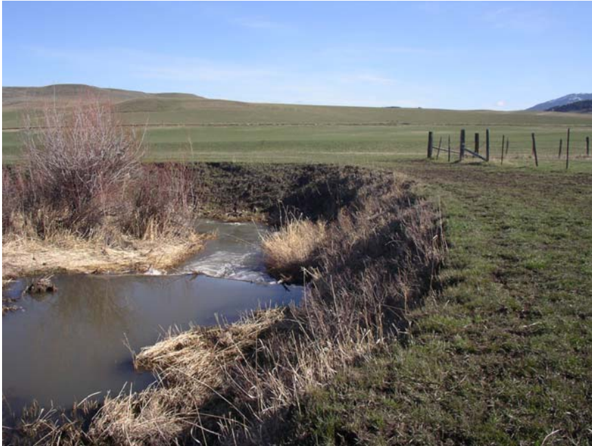
Figure 4-5: Eroding bank stabilized with application of cobble sized rock at the bank's toe.
