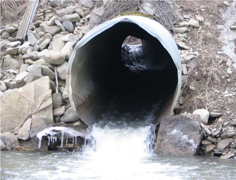
Figure 4-1: Culvert presenting a probable fish barrier on the lower end of the Brumfield property.
