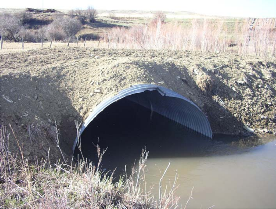
Figure 4-2: New culvert crossing one of the forks of Horse Creek.
