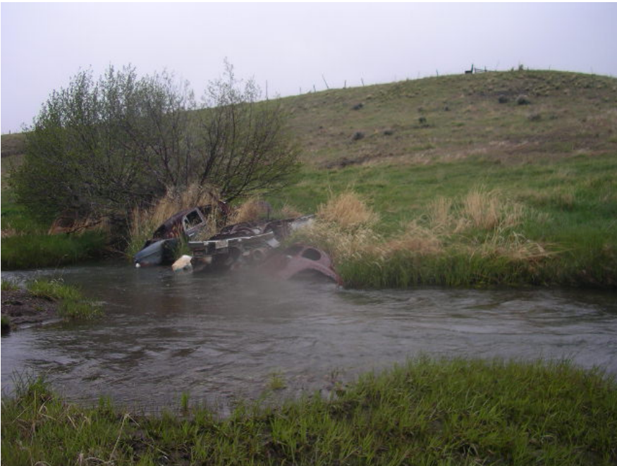
Figure 4-4: Example of car bodies used as bank armor on the lower portion of Brackett Creek on the Lazy S Ranch.
