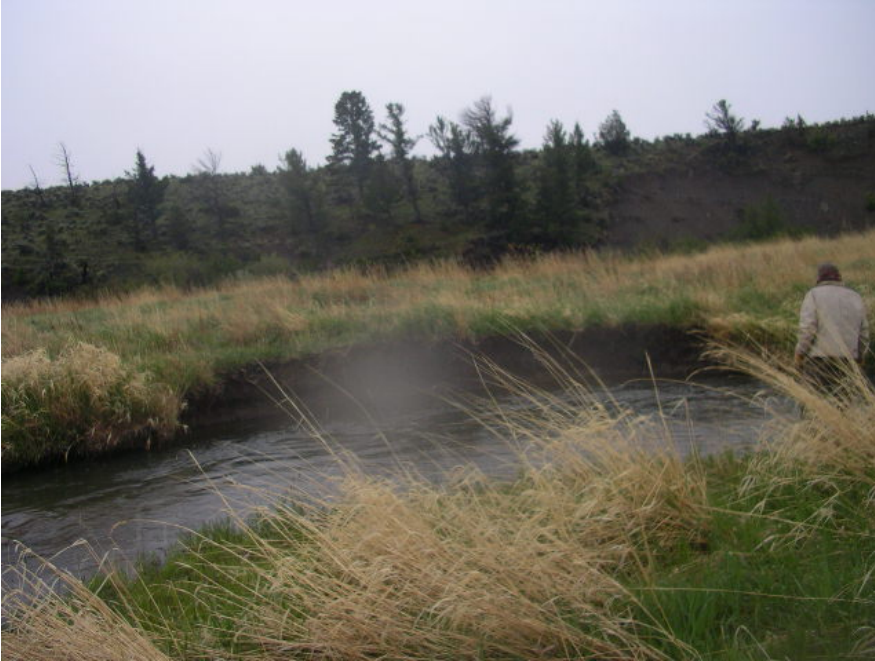
Figure 4-2: Example of localized bank erosion in the constructed channel related to the flood event that occurred in the spring following construction.
