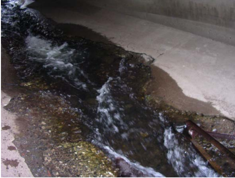
Figure 4-3: Remnant of fish ladder in culvert under the abandoned railroad grade.
