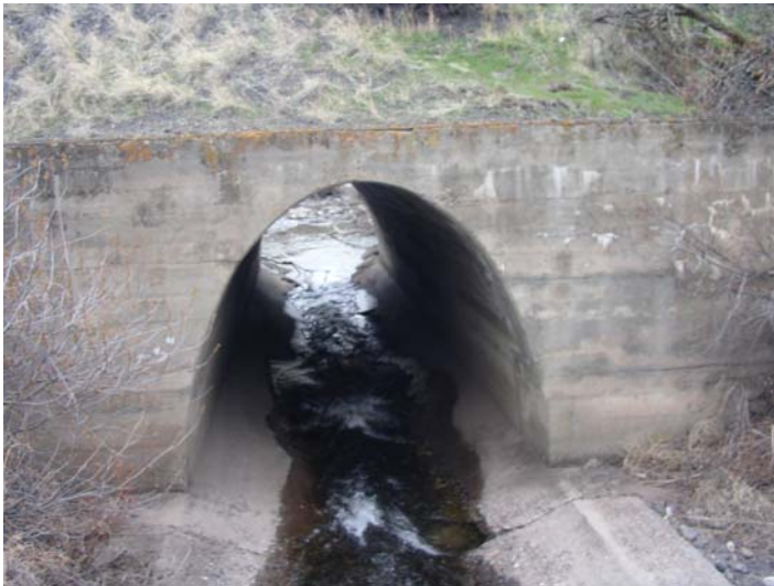
Figure 4-2: Concrete culvert under abandoned railroad grade over Rock Creek.
