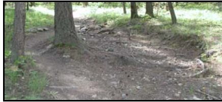
Trail braiding and erosion at Lone
