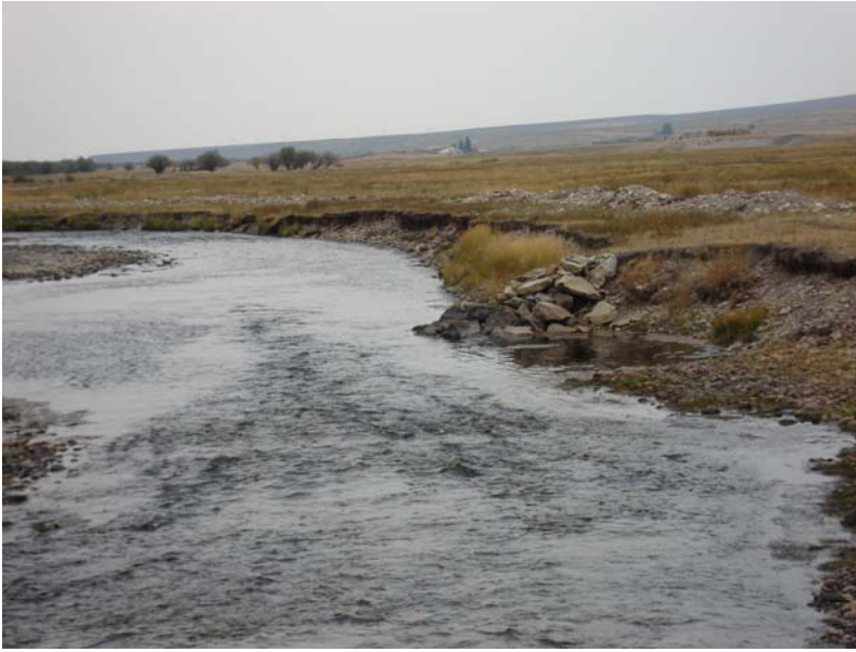
Figure 8. Existing conditions within the Big Hole Restoration – Little Lake Creek Road Reach Project Area.
