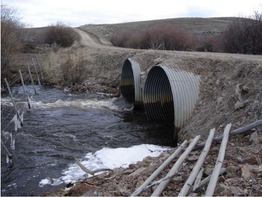
Figure 11. Culverts scheduled for removal in Governor Creek.
