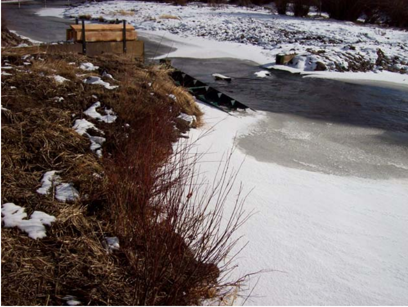
Figure 12. Fish ladder installed in a diversion on Governor Creek.
