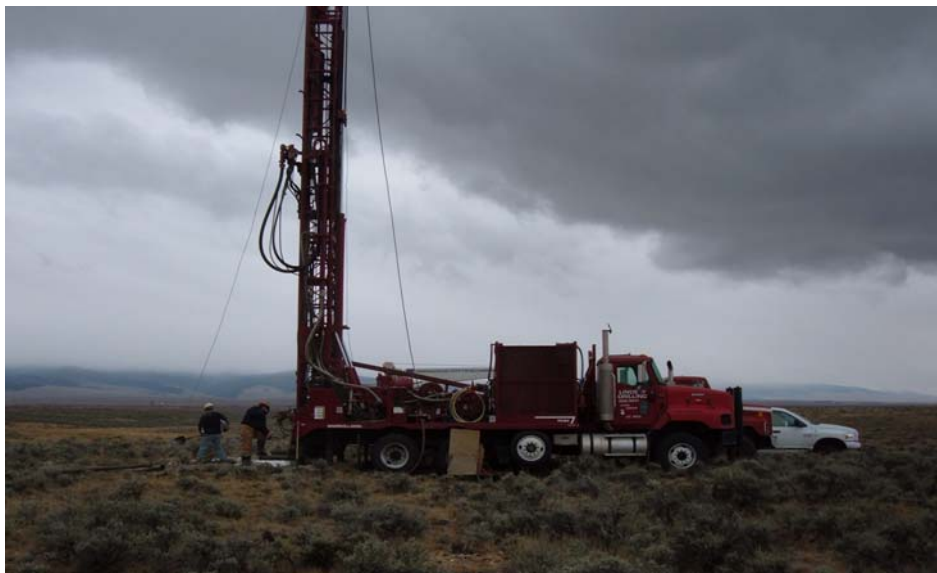
Figure 23. Drilling a stockwater well in the upper Big Hole watershed (project photo).
