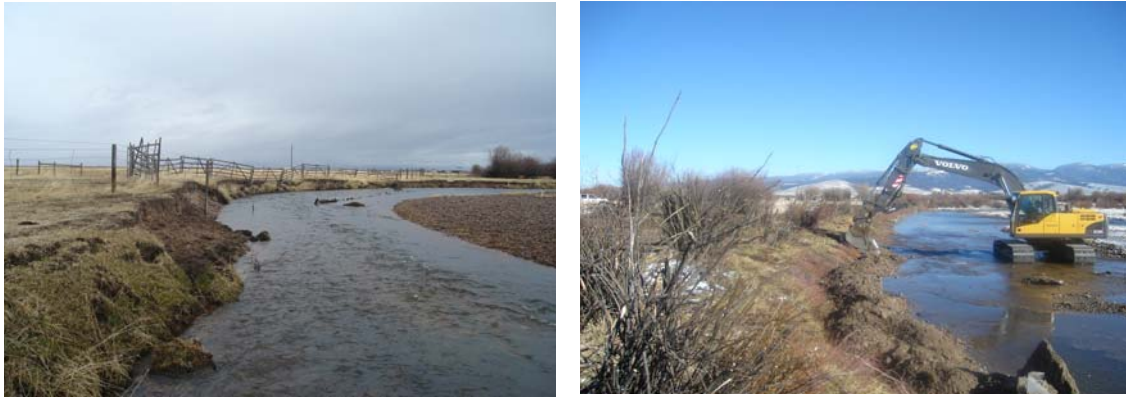
Figure 9. Streambank within the Big Hole River Restoration – Wisdom Reach project area being stabilized with native vegetation and streambank toe armoring techniques (project photos).
