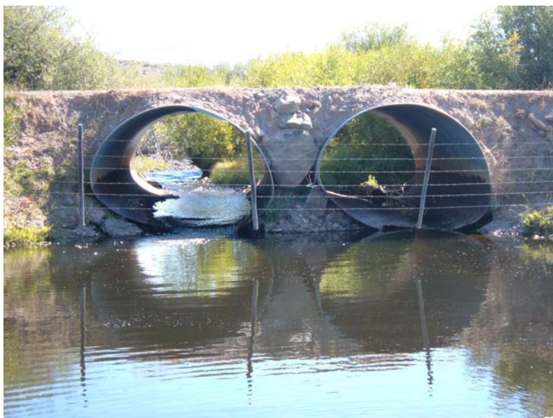
Figure 25. Culverts scheduled for removal in Governor Creek.
