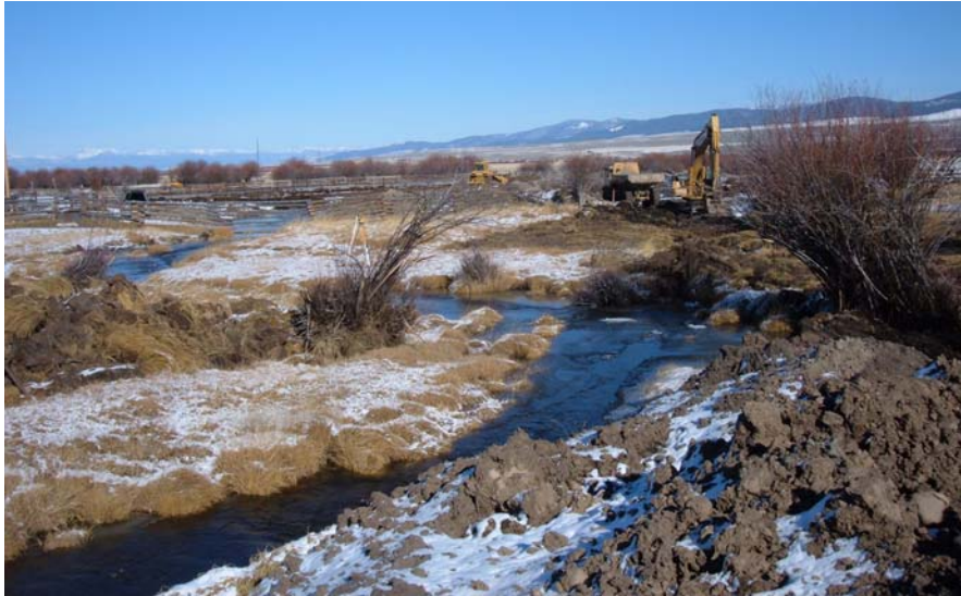
Figure 27. The old stream channel (left) flows through the feedlots in the background, with the restored stream channel under construction to the right.
