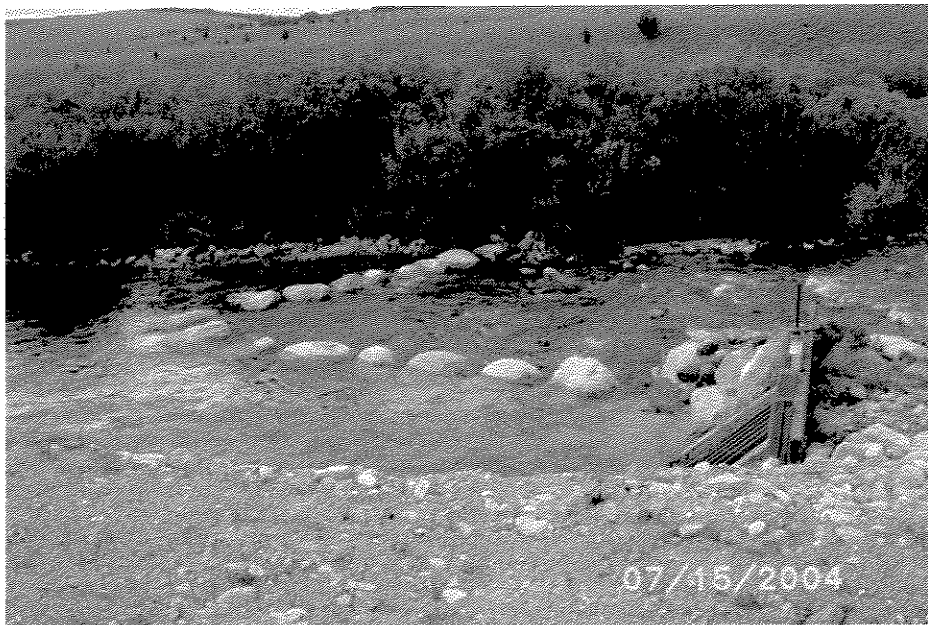
Photo 4G. The proposed diversion structure to replace and improve the current push up diversion structures found on the enrolled land of Landowner “A.” This “rock-vane” diversion is self-sustaining (no streambed disturbance apart from installation) and allows fish passage.
