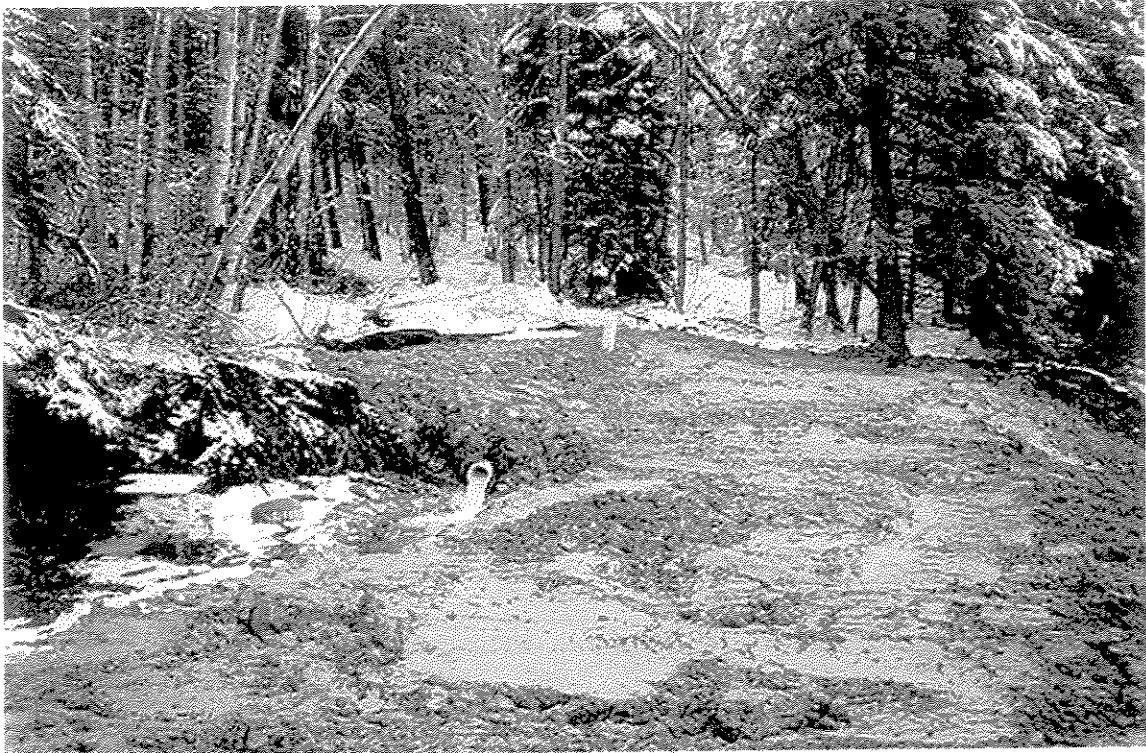
Figure 10. Spring #2 shortly after the spring cap was installed, prior to revegetating the site.
