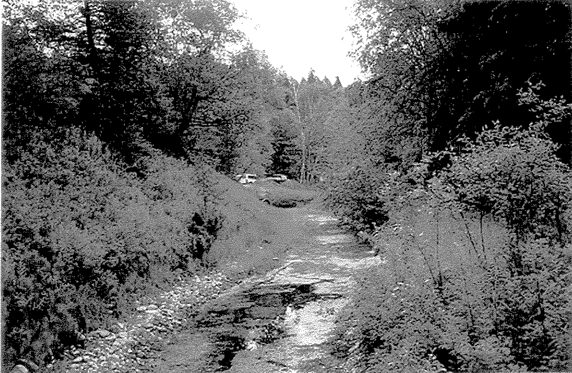
figure 9. Existing linear pond that will become a type E channel extending downstream to type A cascade at the fish viewing window #1. Stream restoration will be accomplished under dry conditions by routing water through a bypass channel that was constructed by the previous owner.
