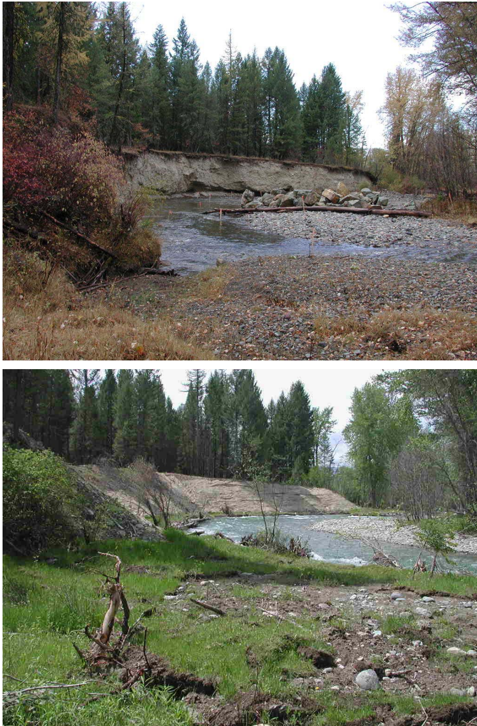
Figure 14. The top photograph shows the lower portion of the Grave Creek Demonstration Project prior to project initiation. The lower photograph shows the lower portion of the restoration project after project implementation. Note the constructed terrace and stream structured in the lower photograph designed to direct stream flow away from the large eroding bank. The project also decreased the slope of this bank and seeded it with grass.
