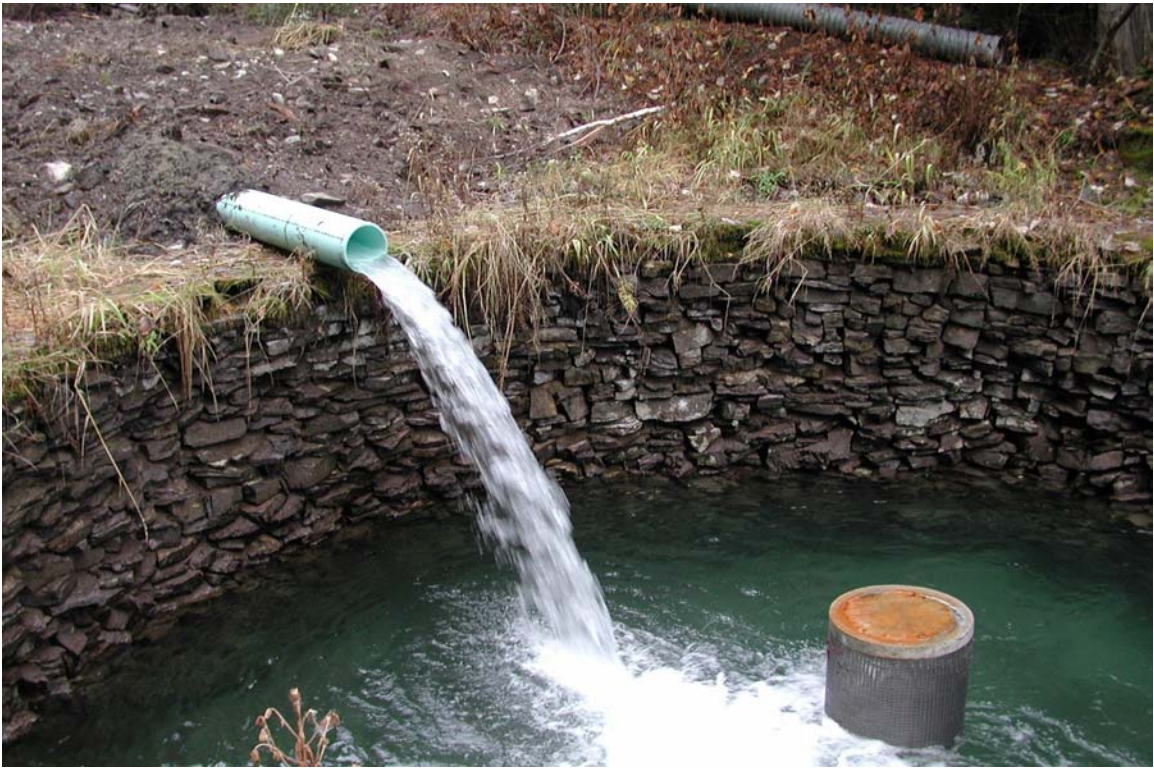
Figure 49. Troy water cistern O'Brien Creek, after change in diversion and installation of new outlet pipe screen cover.
