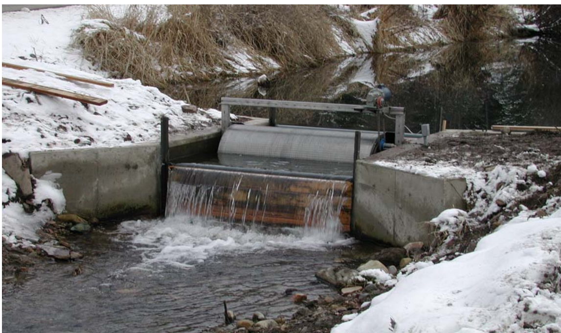
Figure 52. Fish screen at Libby Field Station spring pond, Libby, MT.
