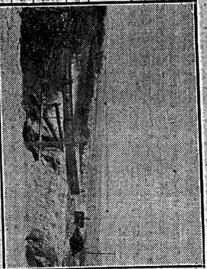
Sun river water pushes through this centrifugal pump made in the drain area and a small lift pump installed to take water to a shelterbelt by the buildings. This pump has a 3-inch suction pipe and a 2 1/2-inch discharge. The farmers had 23 acres in alfalfa last year
