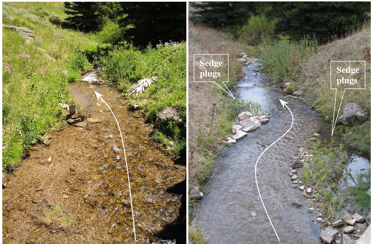
Figure 1. Wigwam Creek immediately downstream of the FS Road 290 bridge; previous to baffle installation (July 2005) at left, and after baffle installation (September 2006) at right.
