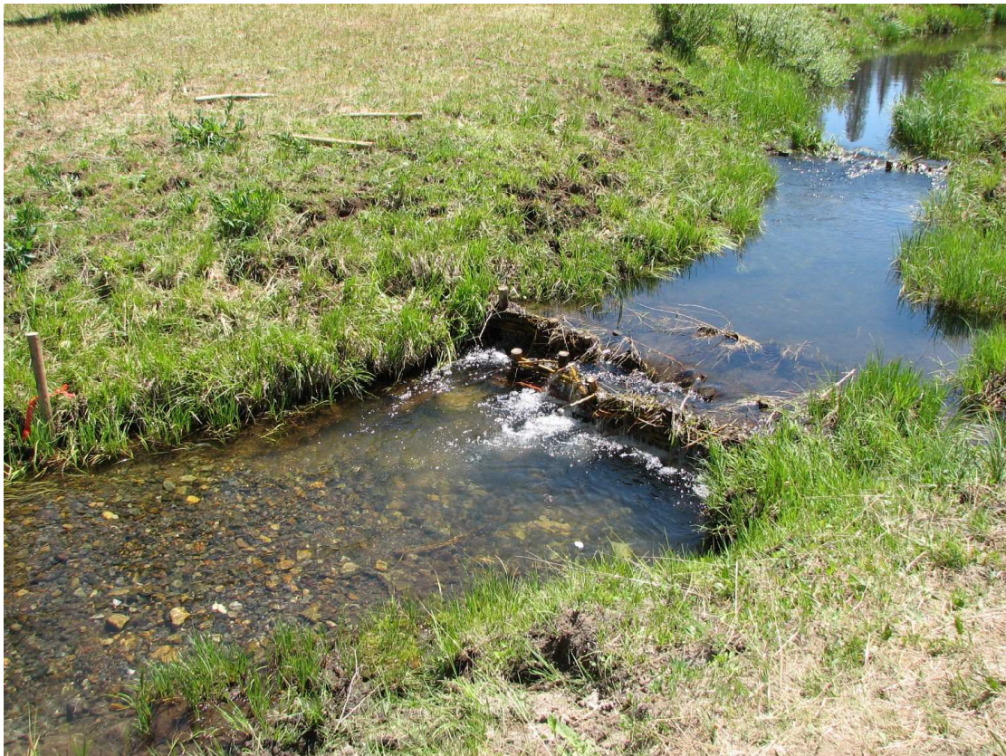
Gazelle Creek, channel spanning structures raising stream bed elevation, August 2007.
