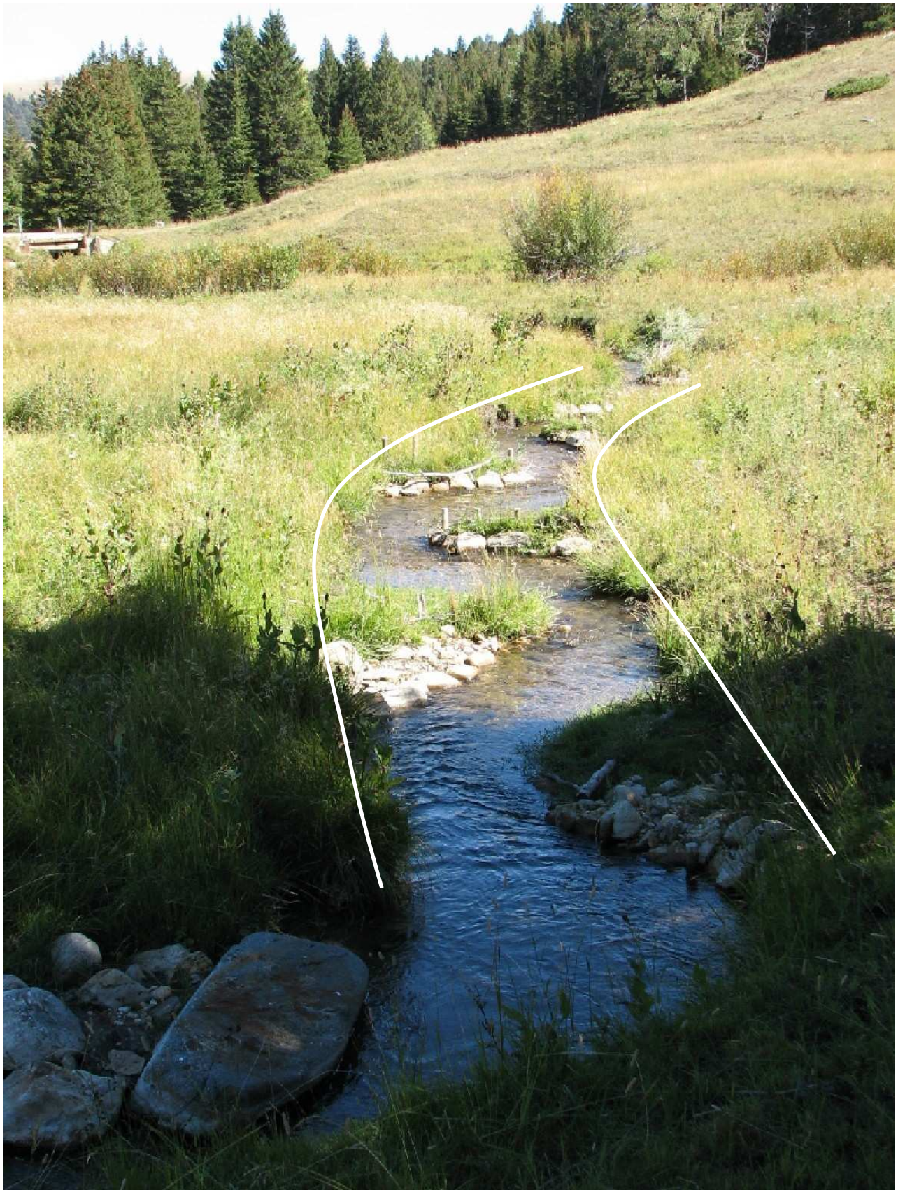
Figure 3. Restored channel segment of Wigwam Creek upstream of the bridge. White lines approximate the pre-treatment location of channel banks. Note how structures have reduced channel width and increased sinuosity. The large rocks at lower left were embedded at the outside bend (at right) of the channel, preventing lateral pool scour and leading to channel straightening. Re-locating these rocks (manually) to the inside of the bend has influenced sediment deposition, point bar formation, and lateral pool scour.
