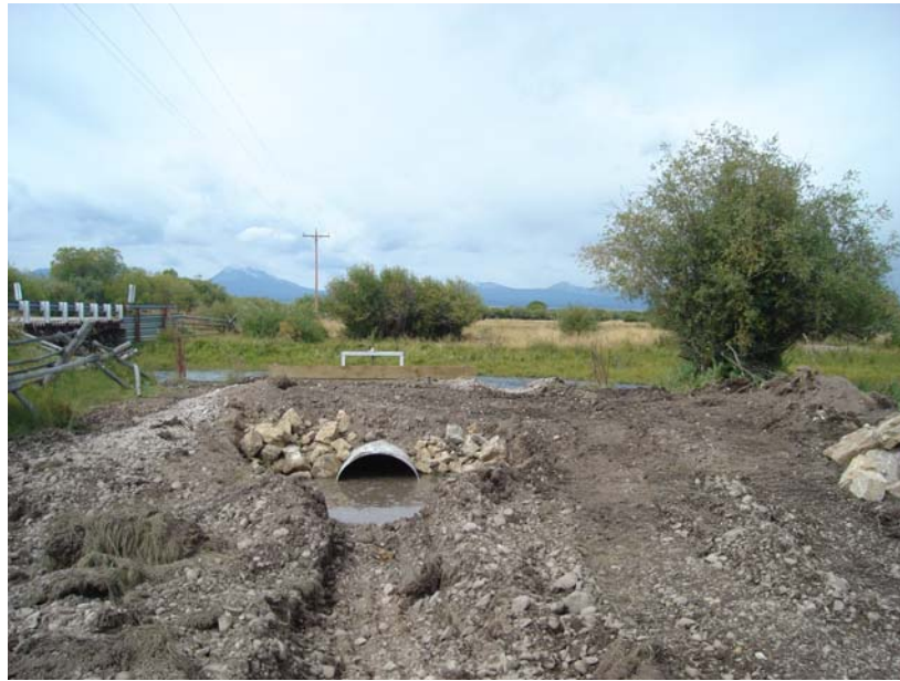
Figure 10. Connecting the new headgate to the irrigation ditch on the Hirschy Irrigation Improvement Project.
