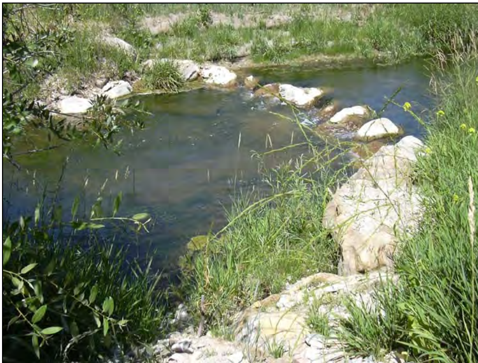
Figure 2-2. Porous Weir on the San Pitch River.
