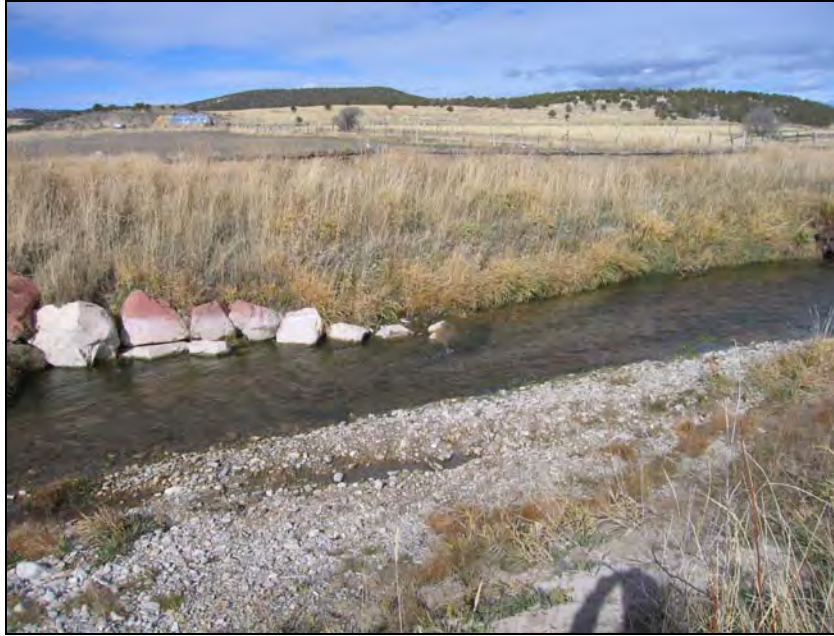
Figure 2-5. Vane on the San Pitch River.
