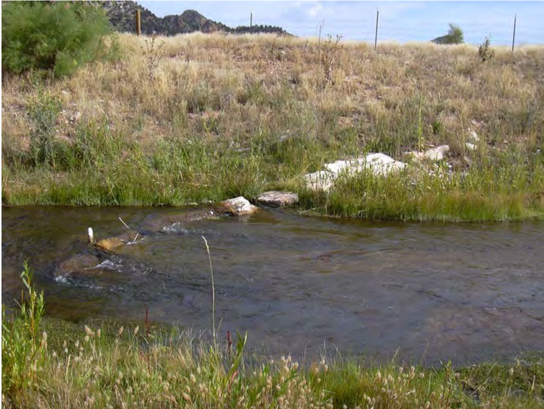
Figure 3-4. J-Hook Structure Observed and Modeled.
