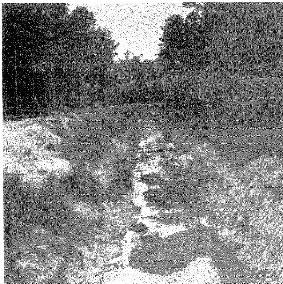
A "Redfin-Warmouth" stream after some stabilization of the ditch.
