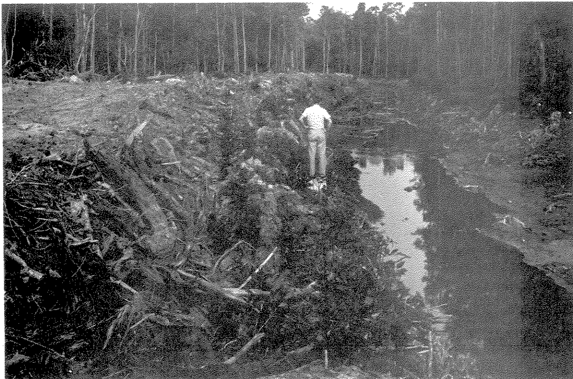
A "Redfin-Warmouth" stream immediately following channelization.
