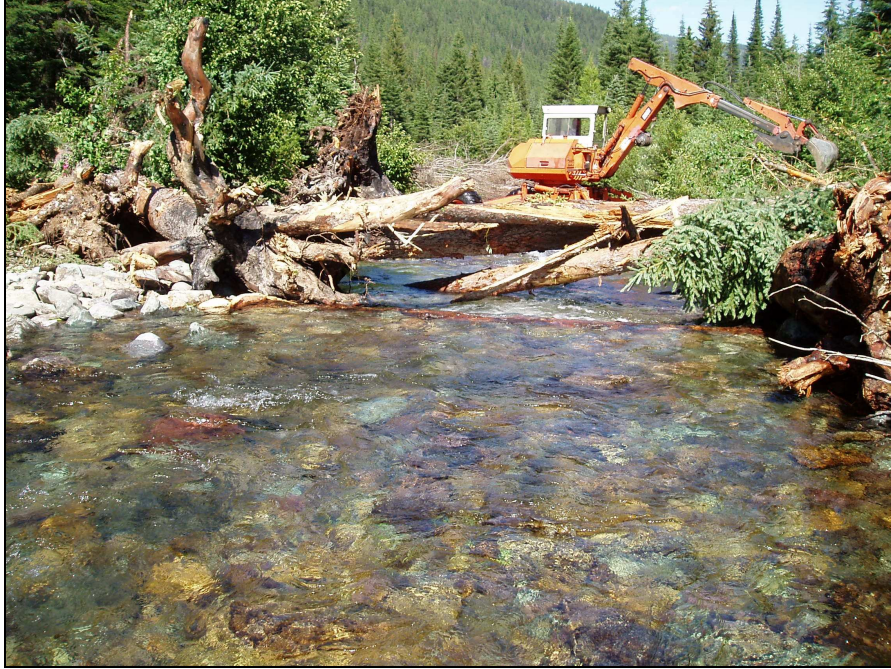
Figure 24. Spider backhoe creating large woody debris aggregate in South Fork Coal Creek during summer 2008.
