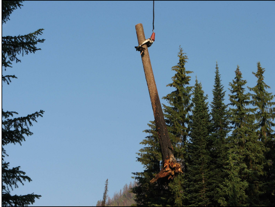
Figure 20. Helicopter placing tree at restoration site location on South Fork Coal Creek in summer 2008.
