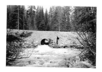
Figure 9 Riverside Greek - Outfall at high water.
