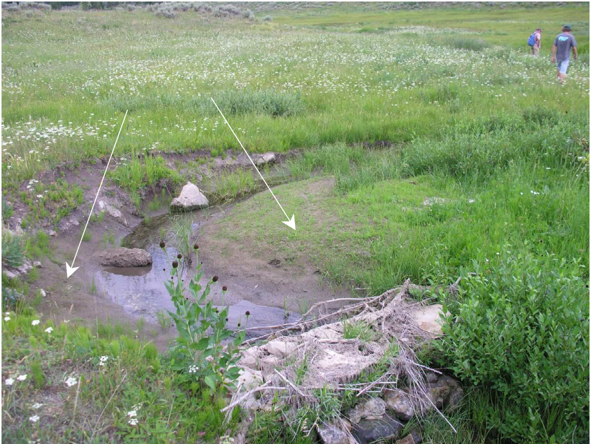
Figure 1. Riffle structure trapping fine sediments upstream (arrows), 2007.
