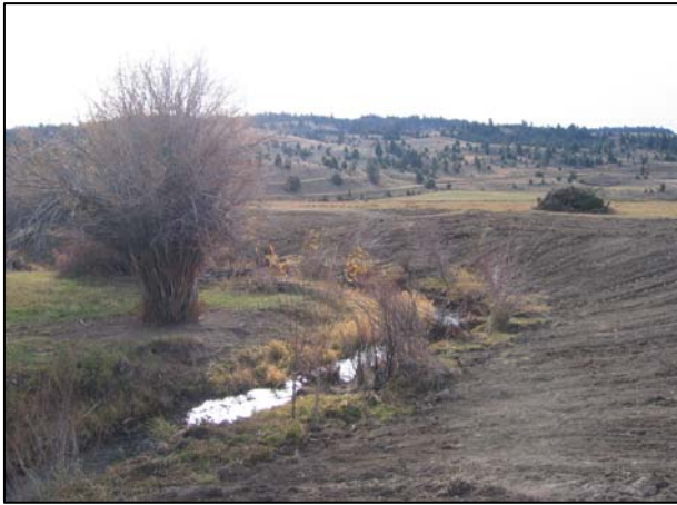
Re-sloping banks on Lazyman Creek allow flows to access the floodplain
