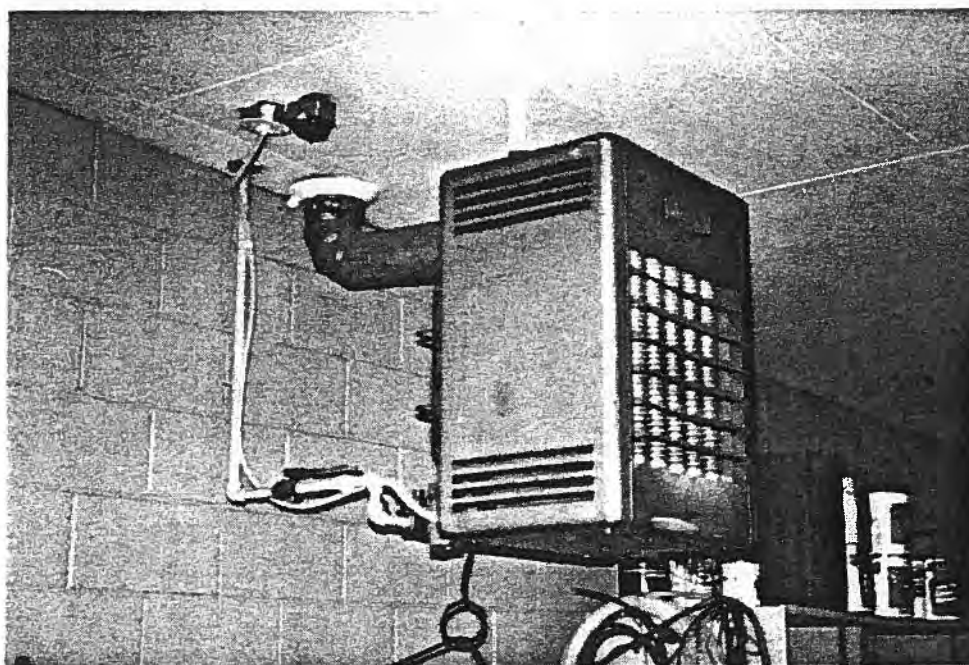
FIGURE 18 MILES CITY SFH - MAIN BUILDING - GAS FURNACE & GAS UNIT HEATERS
