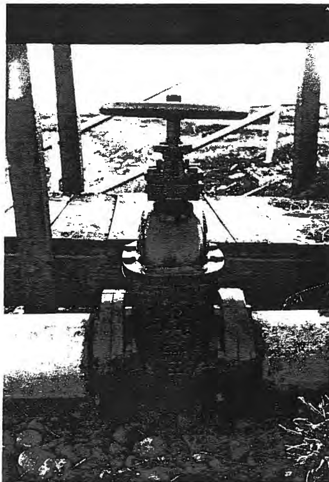
FIGURE 46 OUTLET STRUCTURE SCREEN GUIDES, SLUICE GATE AND VALVE MAINTENANCE PAINTING
