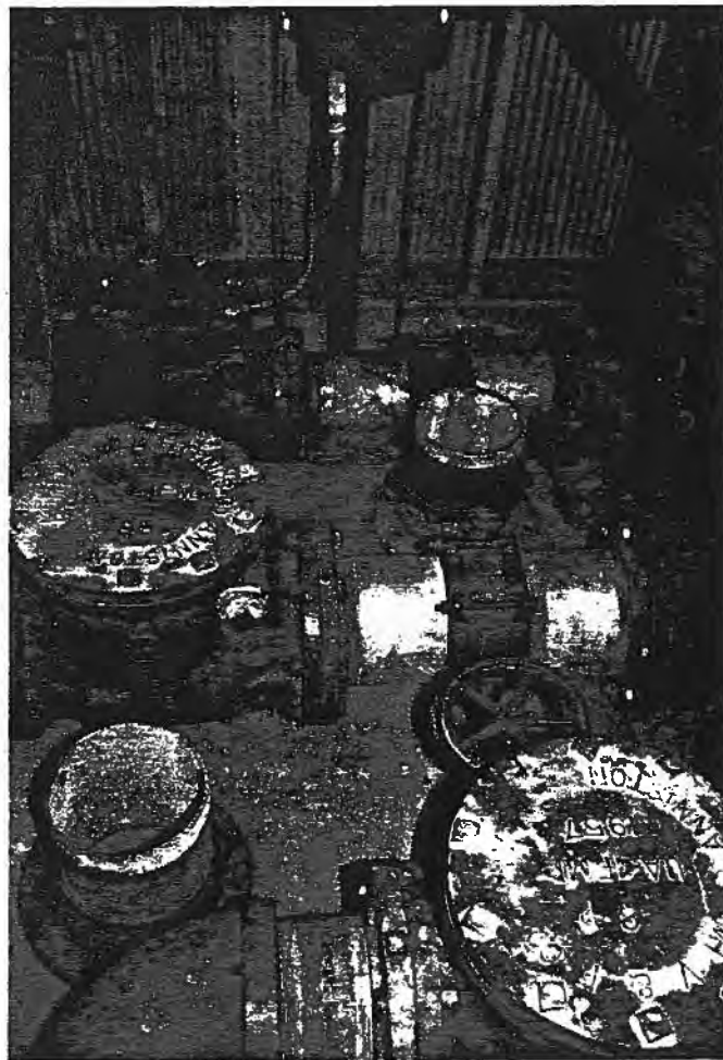
FIGURE 39 REUSE WATER PUMPS AND PUMP CHECK VALVES
