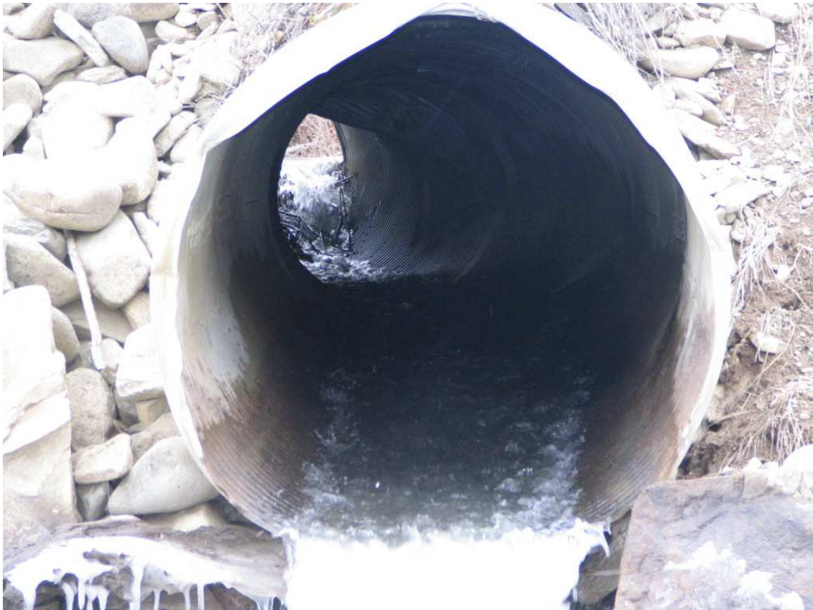
Figure 1-1: Perched, steep, and long culvert on South Fork Horse Creek.
