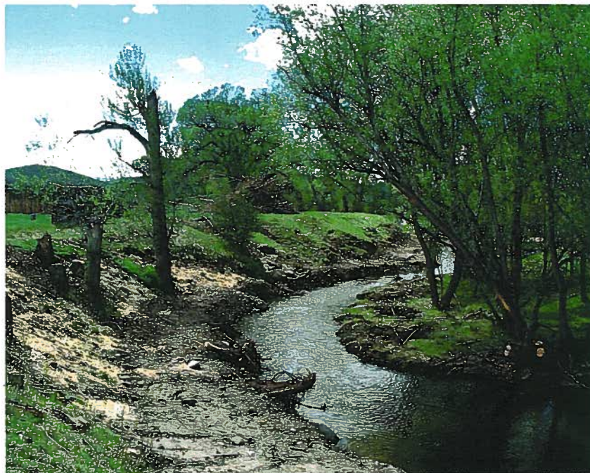
Photo Illustration 1. Restoration of a side channel on the Stillwater River located near the town Absarokee. This abandoned side channel was restored to provide additional spawning and rearing habitat for rainbow trout and brown trout. Upper photo shows side channel during construction. Lower photo shows restored side channel following construction.
