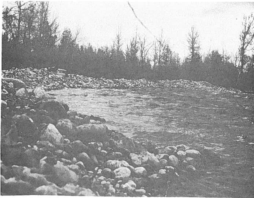
Figure 1. Appearance of stream channel after clearance and realignment work at electric stream census section 3.
