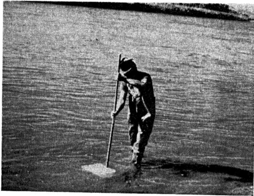
Figure 2. Macroinvertebrate samples were collected with a rectangular framed kick net positioned on the stream bottom.
