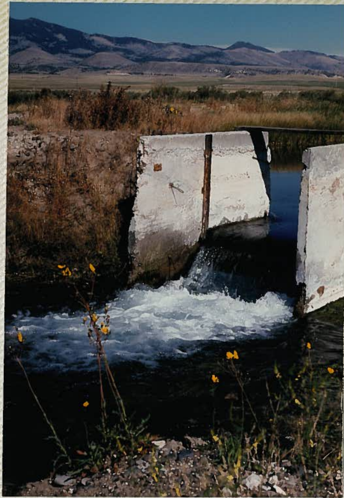
Cold Springs-headgate on upper channel draining ponds.
