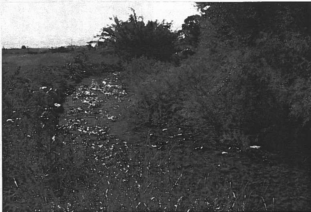
6. A riprapped bend about 1 1/2 years after construction (bend 2, viewed in downstream direction, September 1989). Only the current-bearing (outside) bank is riprapped; stabilizing inner (point bar) banks of bends is unneeded, even where less well vegetated than this--and is unwise from standpoints of cost and fish/wildlife habitat. A common mistake in streambank stabilization, done in the name of fish habitat improvement, is to revet both stream banks, thus often overly constricting the channel, impeding natural processes to which fish are adapted, and destroying or hampering regrowth of bankside vegetation.
