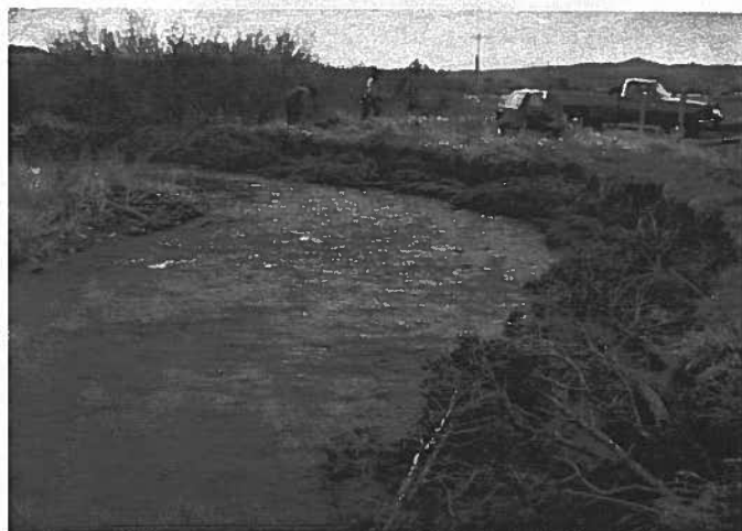
3. Stream bend after trees have been anchored.
