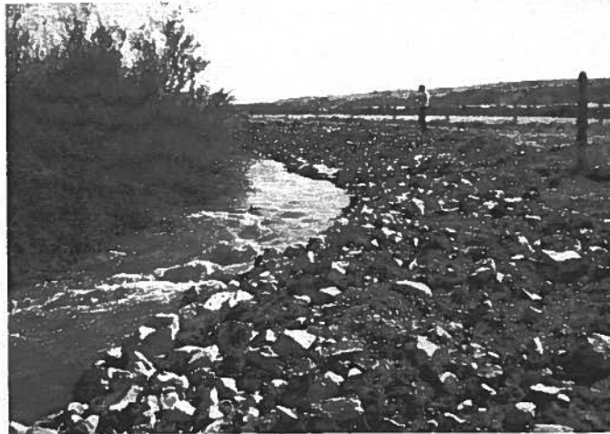
5. Finished riprap (bend 16).
