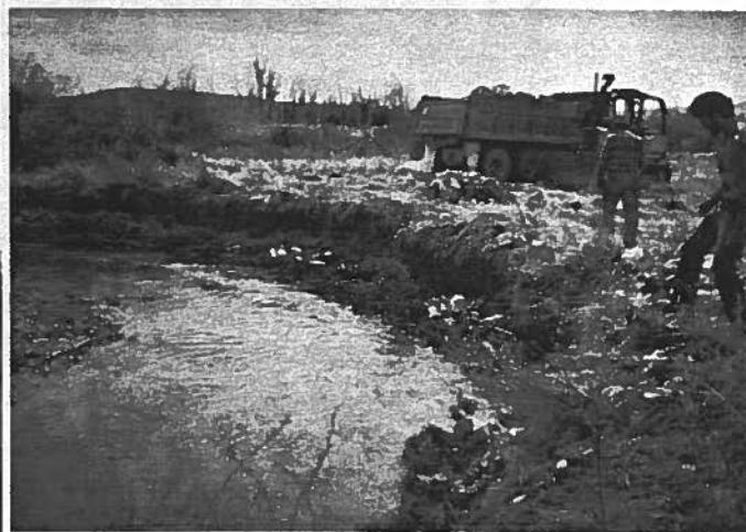
4. Backfilling with field rock.
