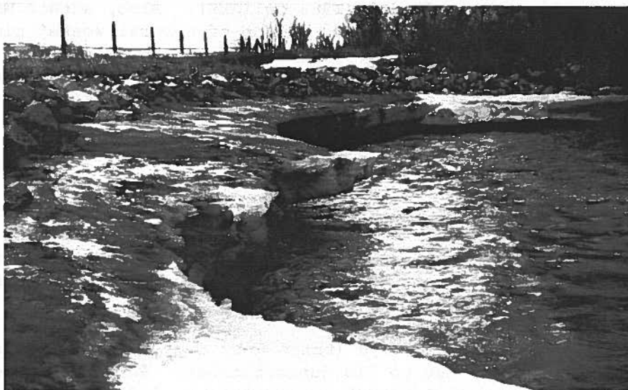
Figure 32. A streambank ice shelf supported by riprap, Deep Creek, Montana, spring 1989.
