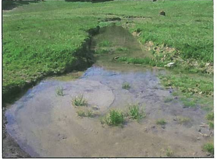
Sediment deposit upstream of weir structure.
