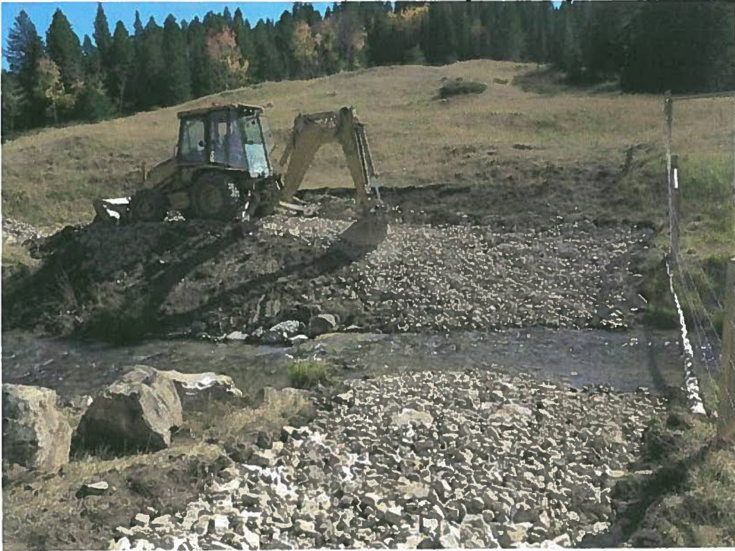
Photo 3. Armored ford construction, note base layer of compacted cobble and gravel.
