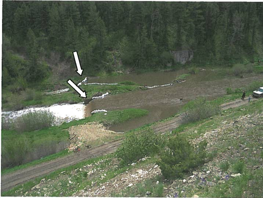
Figure 14. Two barriers, indicated by arrows, separating Cherry Creek phases 3 and 4 during Spring runoff 2010. At the height of runoff and prior to sandbagging, water flowed overland between the two barriers. A retired irrigation ditch is adjacent to the road. Turner Enterprises photo.
