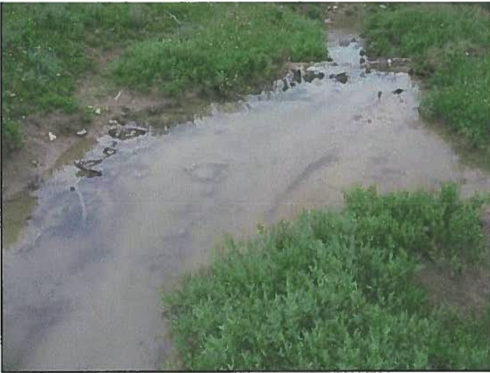
Sediment deposition influencing the main channel after one year.
