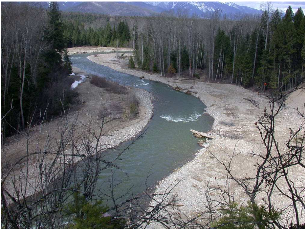
Figure 3. Top photograph shows the largest of the two eroding banks within the Libby Demonstration Project prior to project implementation. The lower photograph was taken after project construction. Note the position of the stream in the upper photograph against the eroding hillside that was over 700 feet long and averaged 80 feet high.
