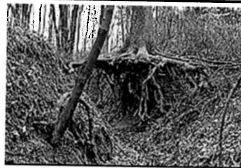
Gully erosion from storm water runoff
