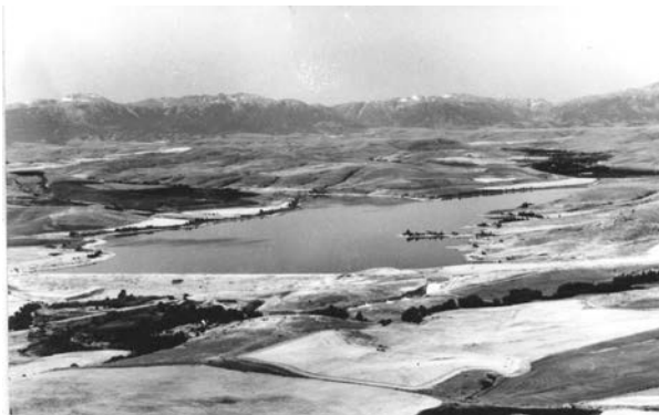
Image 2. Cooney Reservoir after construction of dam. State Water Conservation Board – State Engineers Office, July 1952.
