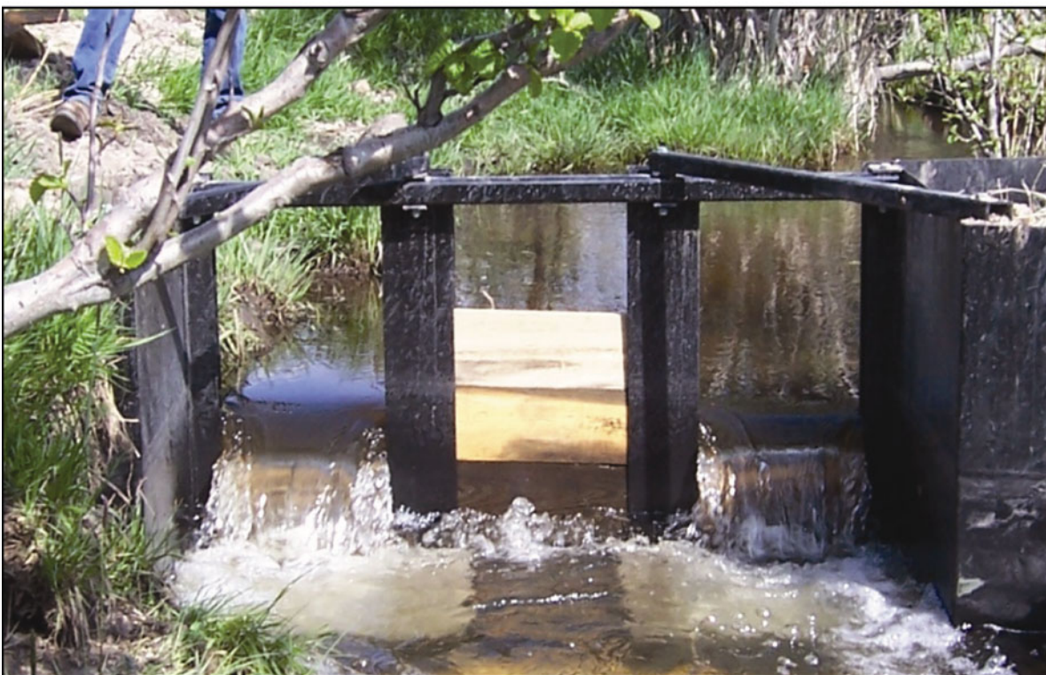
FIGURE 2. Picture of a Coanda diversion and fish screen on Wasson Creek. The photo shows two fish screens as well as a sediment sluice gate (middle slot with boards). The smaller photo (top) shows an adult Westslope Cutthroat Trout ascending the Coanda. (Photo by Jamie Nesbit.)
