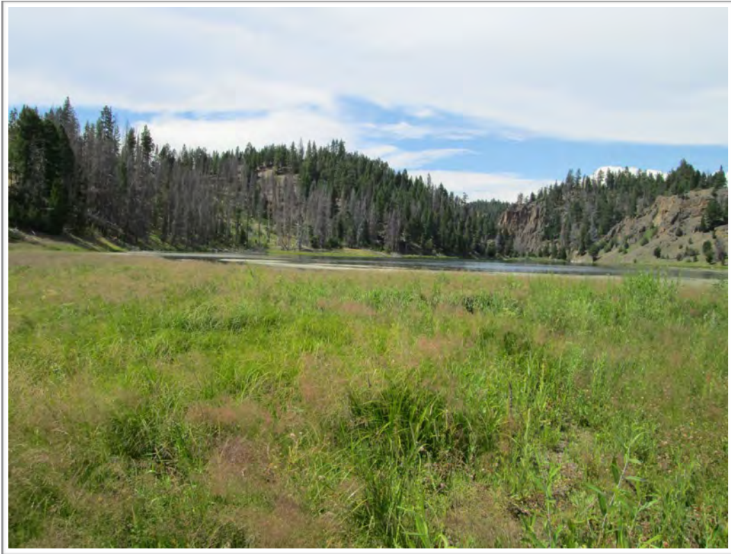
Photo 42. Looking north to the dam on Spotted Dog Reservoir (2014 photo)
