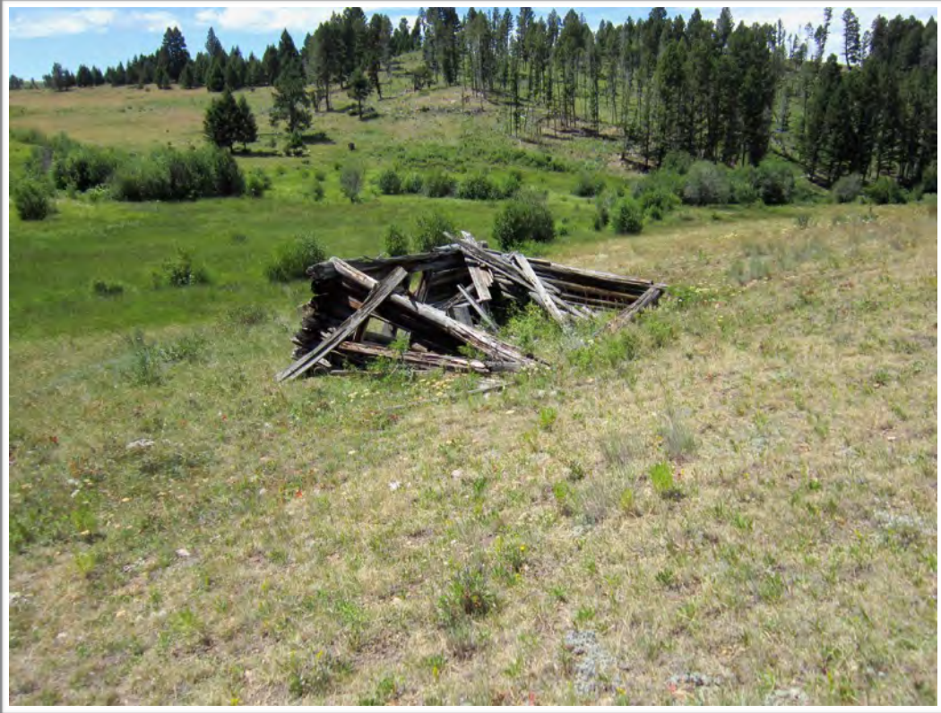
Photo 58. A historic cabin adjacent to an unnamed tributary to Trout Creek (2014 photo)
