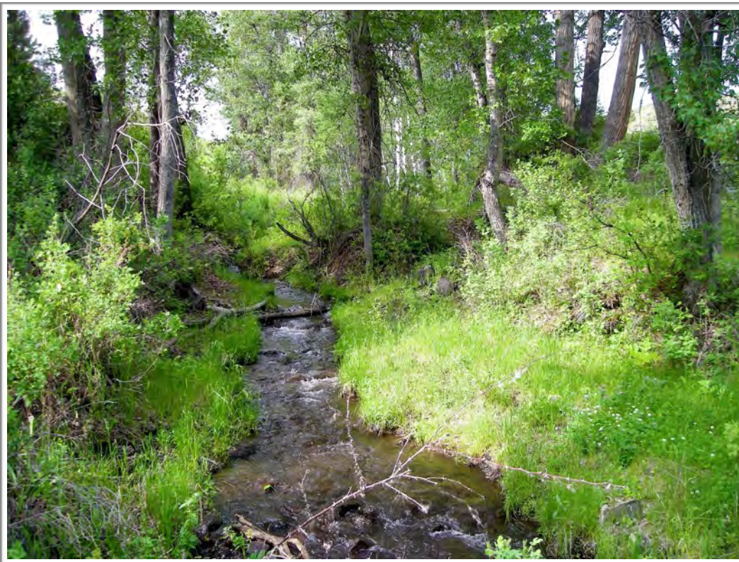
Photo 75. Typical view near the lower end of Freezeout Creek, showing a lack of plants with deep, binding roots along the channel (Record ID 2024181) (2011 photo)
