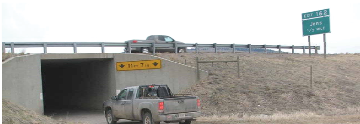
Typical existing underpass for livestock and ranch traffic that may serve for elk someday.
