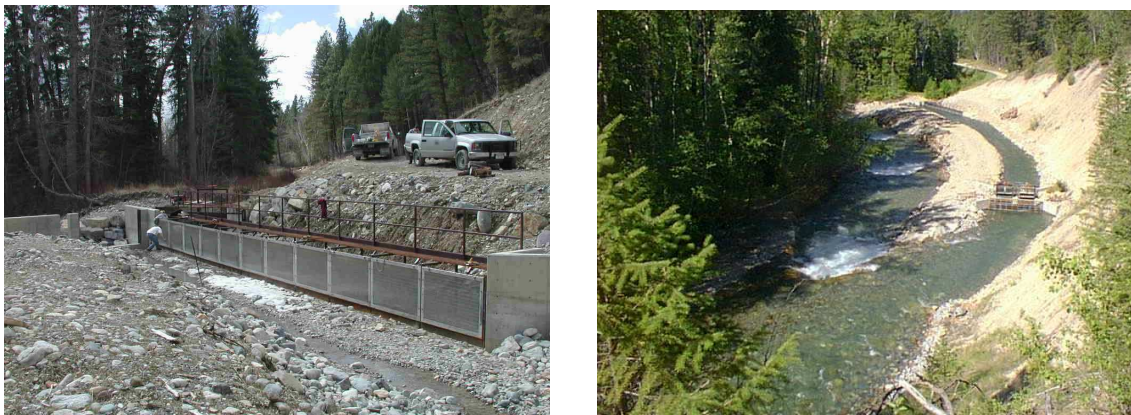
Figure 2. Photographs of Glen Lake Irrigation District diversion on Grave Creek, Montana. Left photo shows passive wedge wire screen, right photo shows diversion with upper headgate and cross vane structures.
