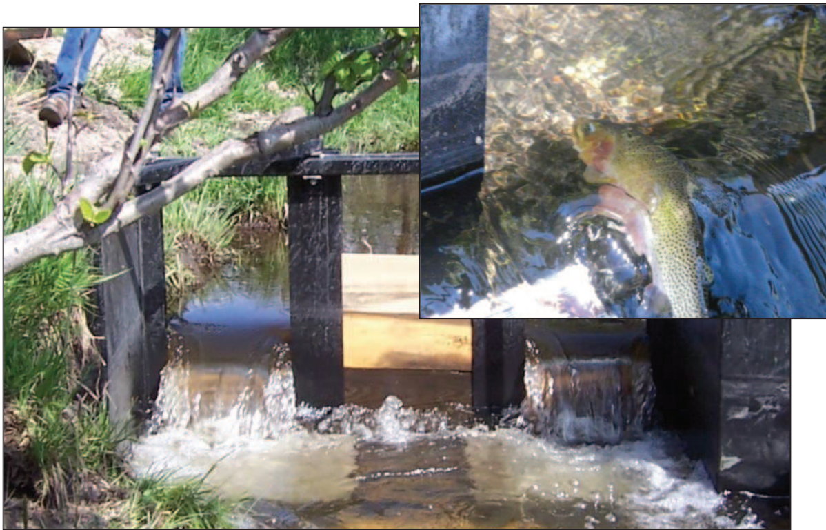
Photo 1a and b. Photo of a Coanda diversion and fish screen on Wasson Creek. The large photo shows two fish screens as well as a sediment sluice gate (middle slot with boards). The smaller photo in the upper right shows an adult westslope cutthroat trout ascending the Coanda (Photo by Jamie Nesbit).
