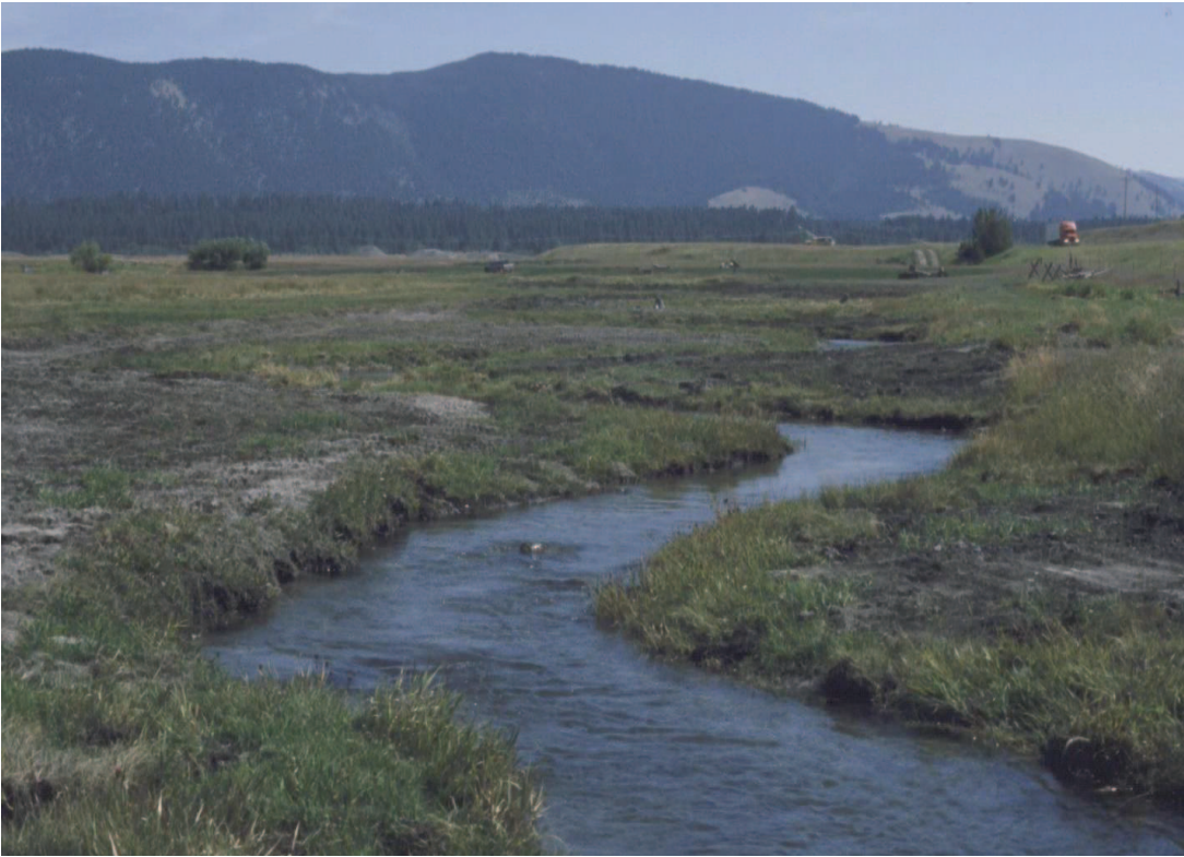
Photos 1 and 2. Kleinschmidt Creek before (top) and after (bottom) restoration in 2001. The top photo shows straightened and widened section of channel with an example of a rock dam that trapped sediment. The bottom photo was taken immediately after channel reconstruction in the late summer of 2001.
