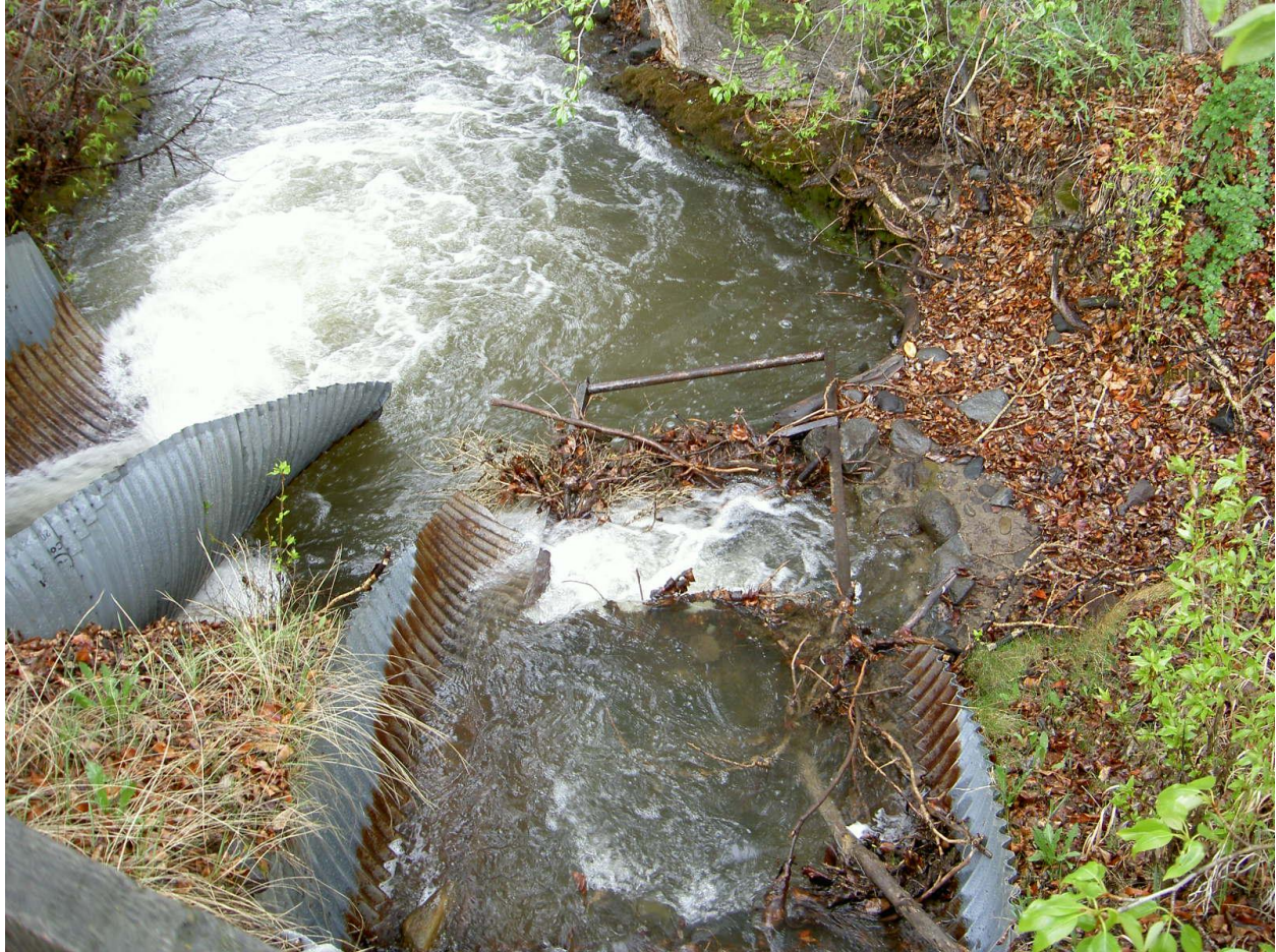
• Figure 2: Downstream end of the two culverts under HWY 89 South. You can see part of the historic fish ladder frame in the culvert on the right. Photo courtesy of Montana Dept. of Transportation.
