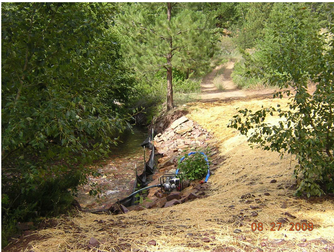
Figure 6. Lyons Creek site with topsoil, seed, straw and trash pump for watering.
