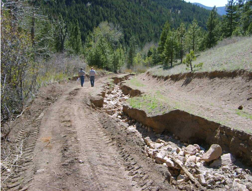
Figure 3. Foster Gulch washout in the center of the main access road approximately 300 yds from the confluence with Little Wolf Creek. July 2009.
