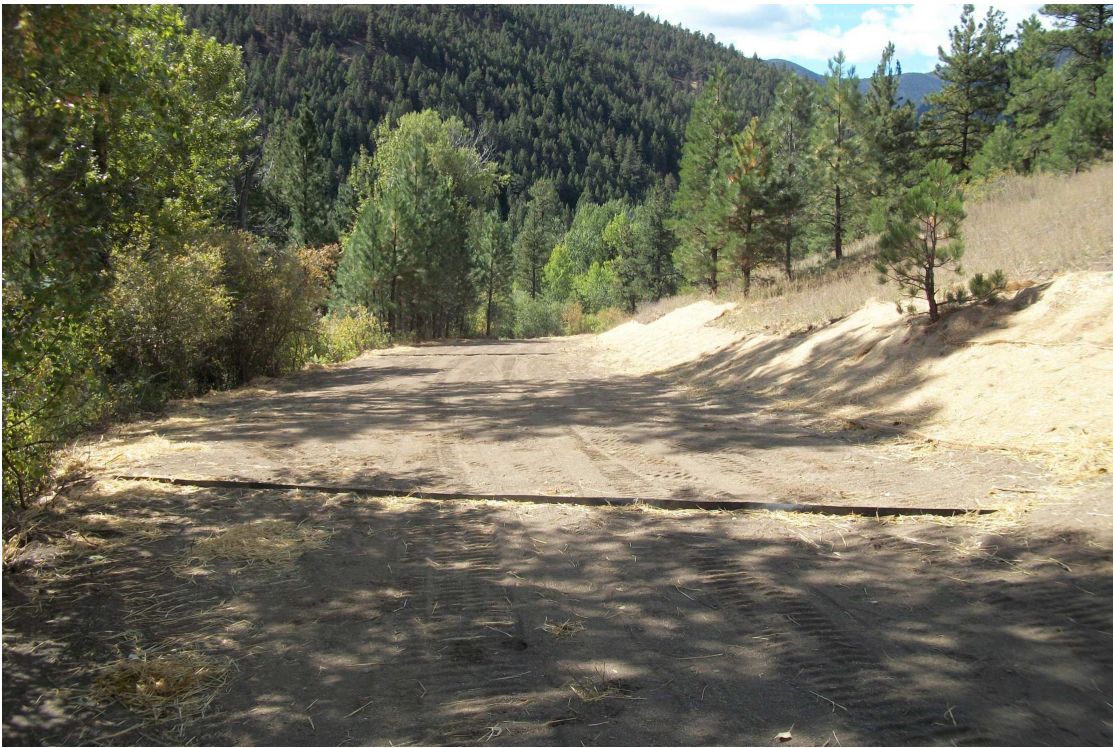
Figure 6. New road grade with wash-out repaired and water bars installed, Foster Gulch October 2011.
