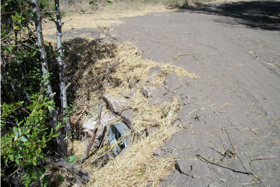
Figure 7. Lower stream crossing after new culvert and BMPs installed. Foster Gulch, October 2011
