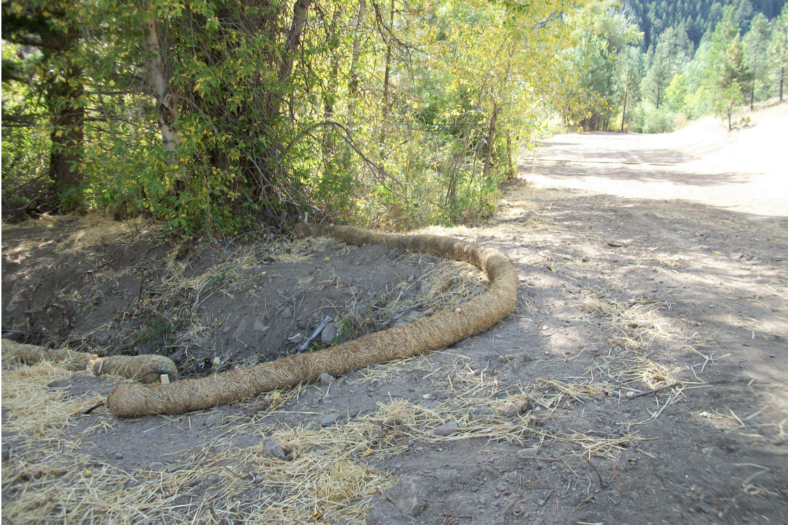
Figure 5. Upper stream crossing after new culvert and BMPs installed. Foster Gulch, October 2011.
