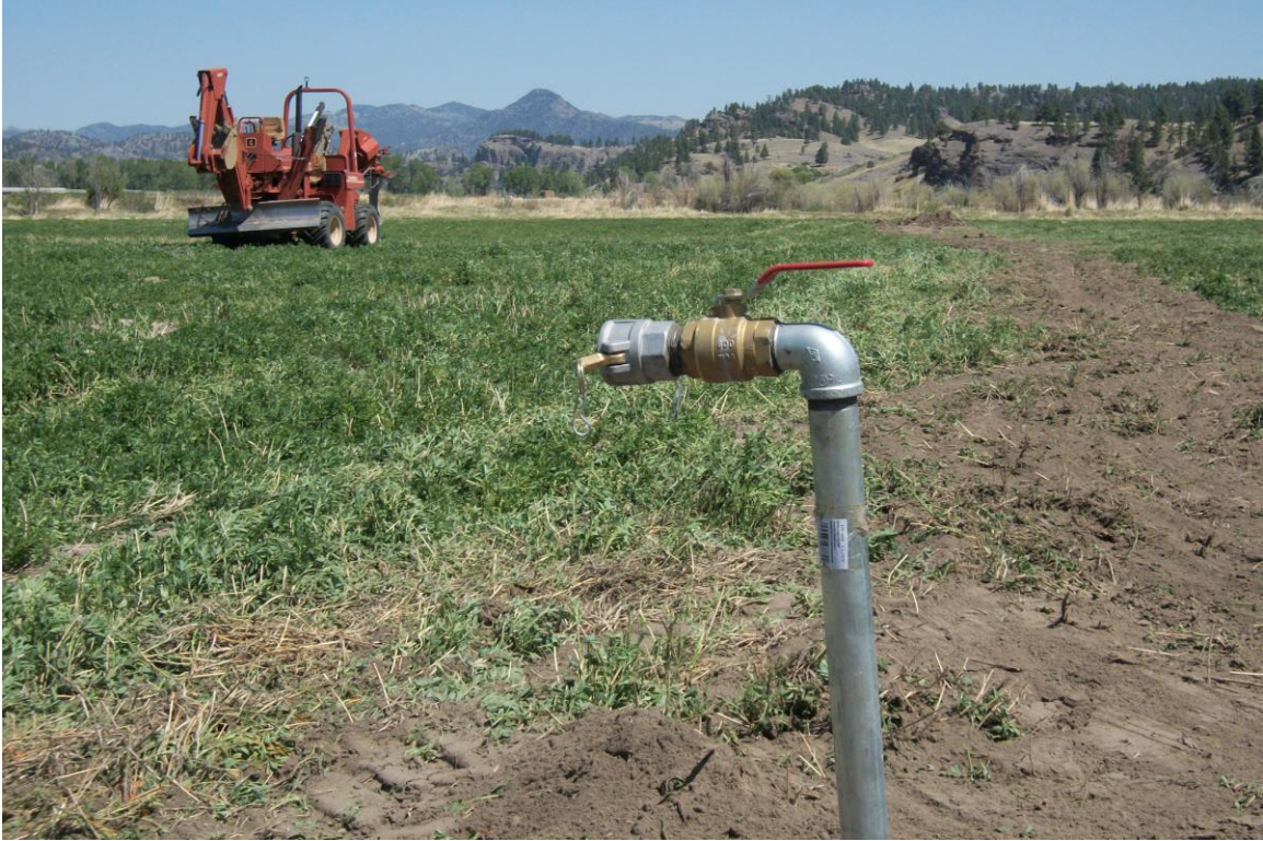
Figure 10. Riser line for livestock water and irrigation at Craig field, Sterling Ranch, Craig Montana 2012.
