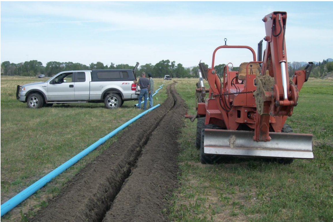
Figure 9. Installing mainline water pipe at Craig field, Sterling Ranch, Craig Montana 2012.
