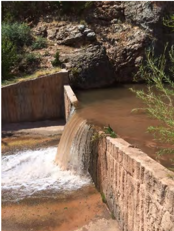
Figure 2-22. View upstream of the face of the weir showing accumulation of cohesive bed load.
