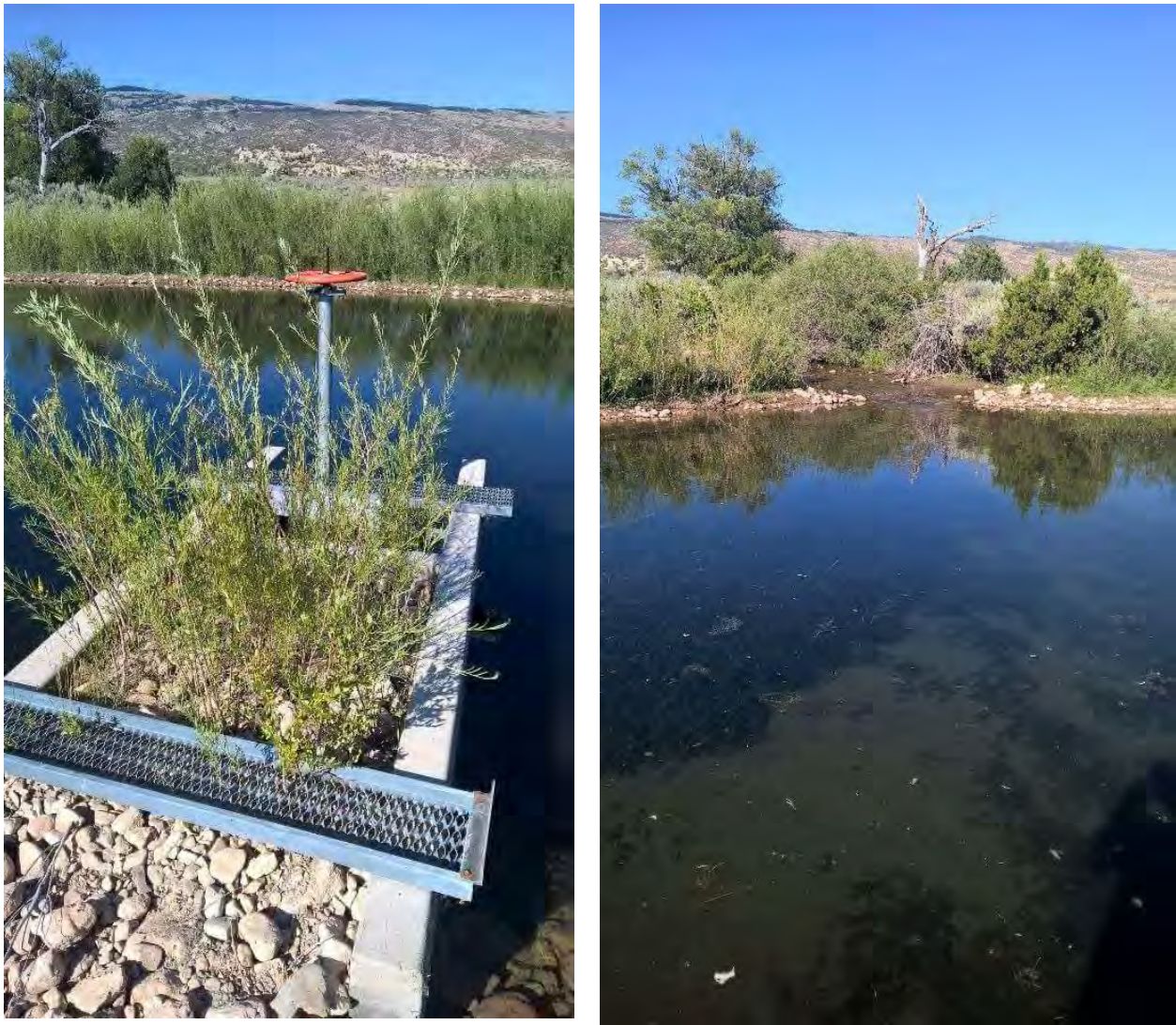
Figure 2-71. Stand pipe diversion, and inlet of Piney Creek into the storage pond.
