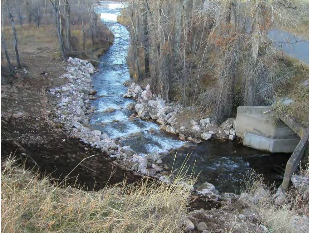
Figure 2-17. Post-construction photo of step-pool sequence providing passage up to, and through, the
