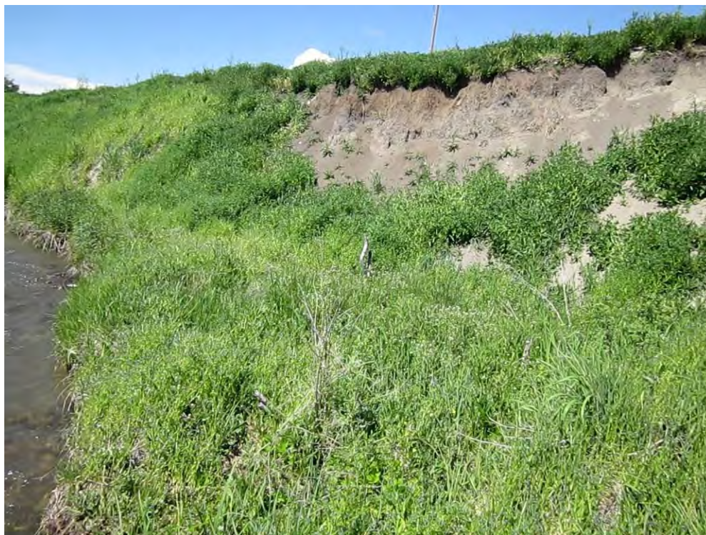
Figure 2-90. Floodplain bench 5 years after construction.
