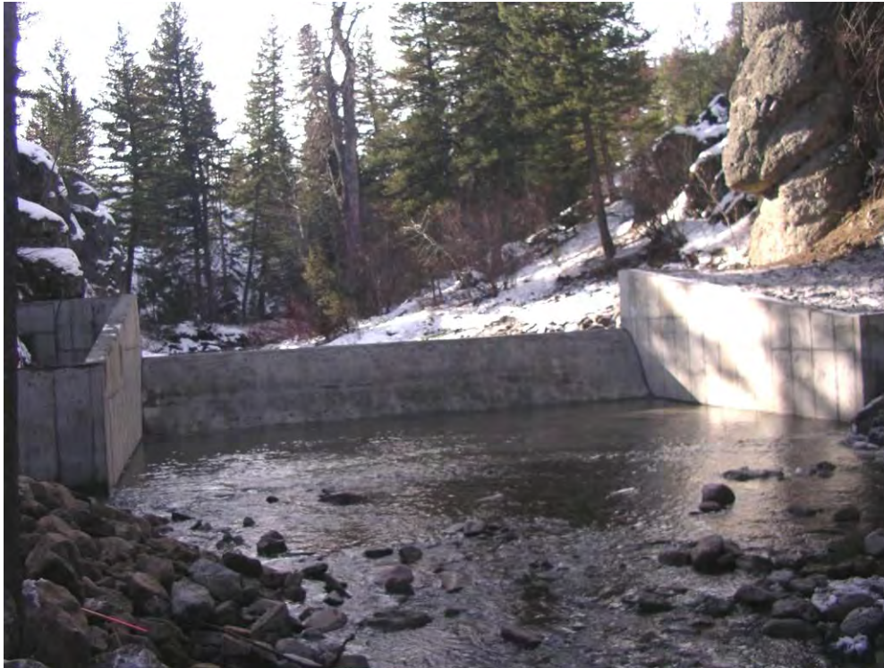
Figure 2-60. Newly constructed barrier on Lower Deer Creek.
