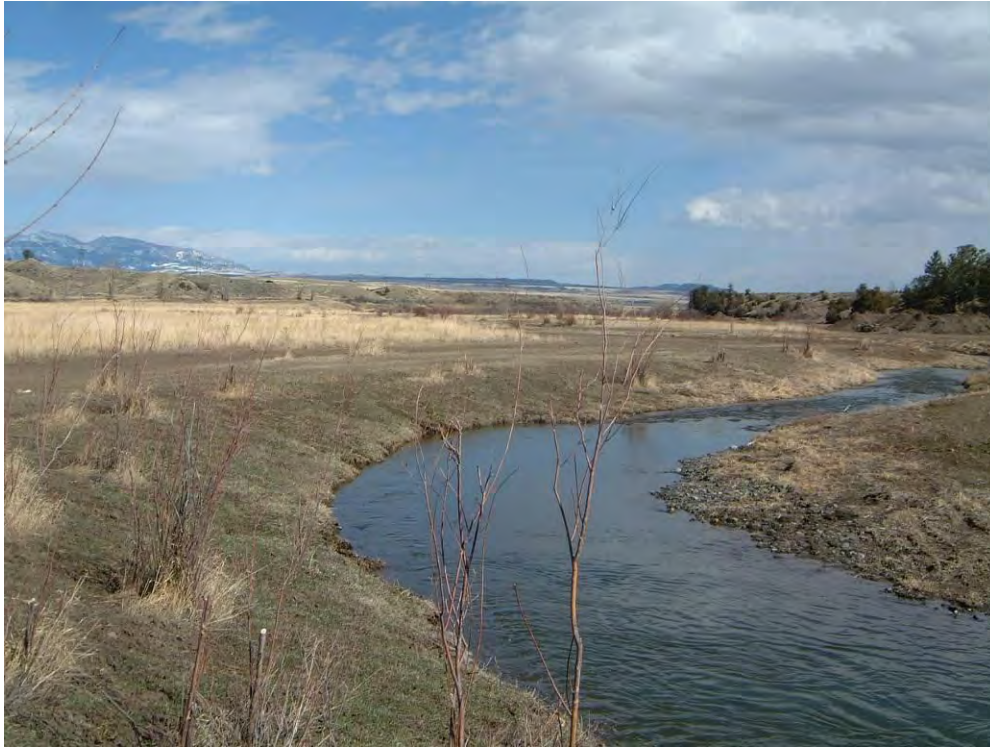
Figure 2-9. Brackett Creek re-naturalization immediately post-construction.
