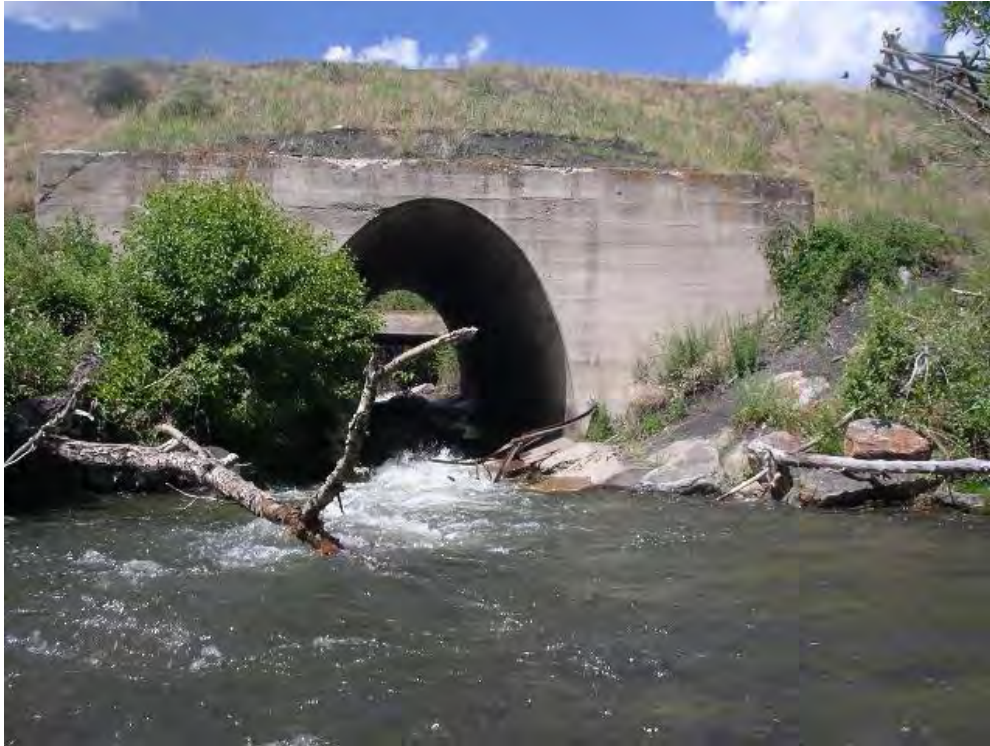
Figure 2-72. Railroad culvert on Rock Creek.
