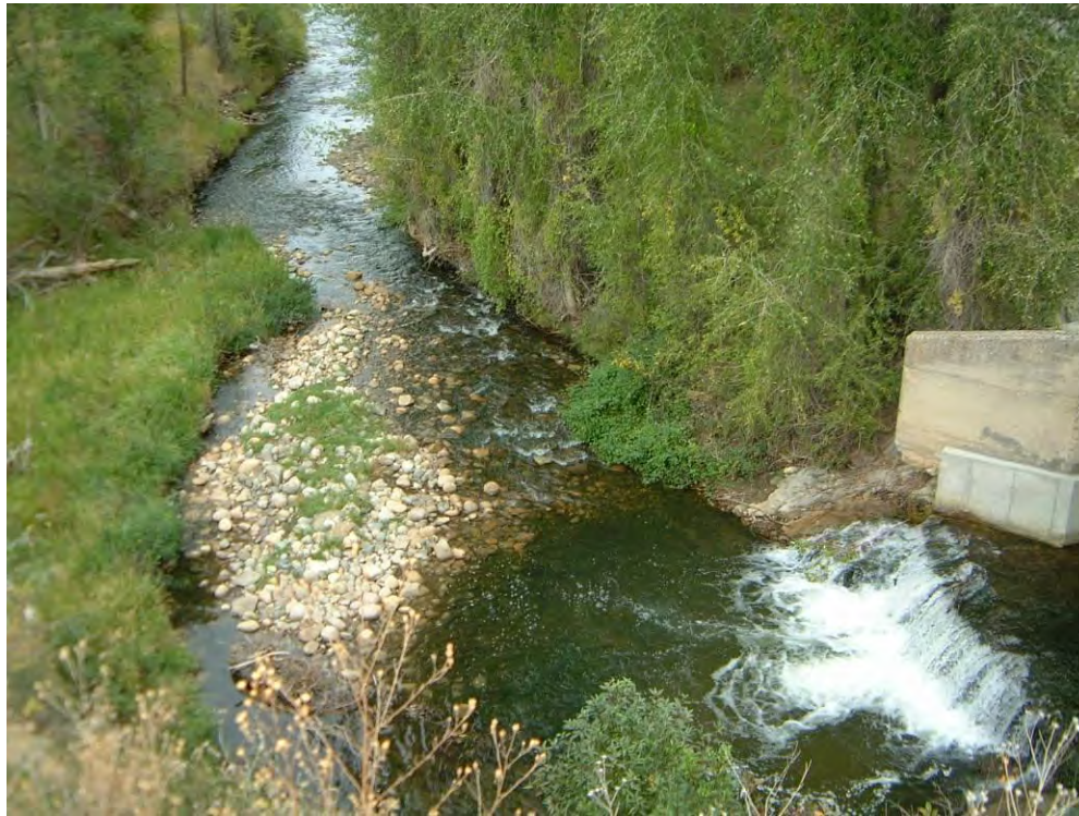
Figure 2-16. Impassible culvert on Clear Creek.
