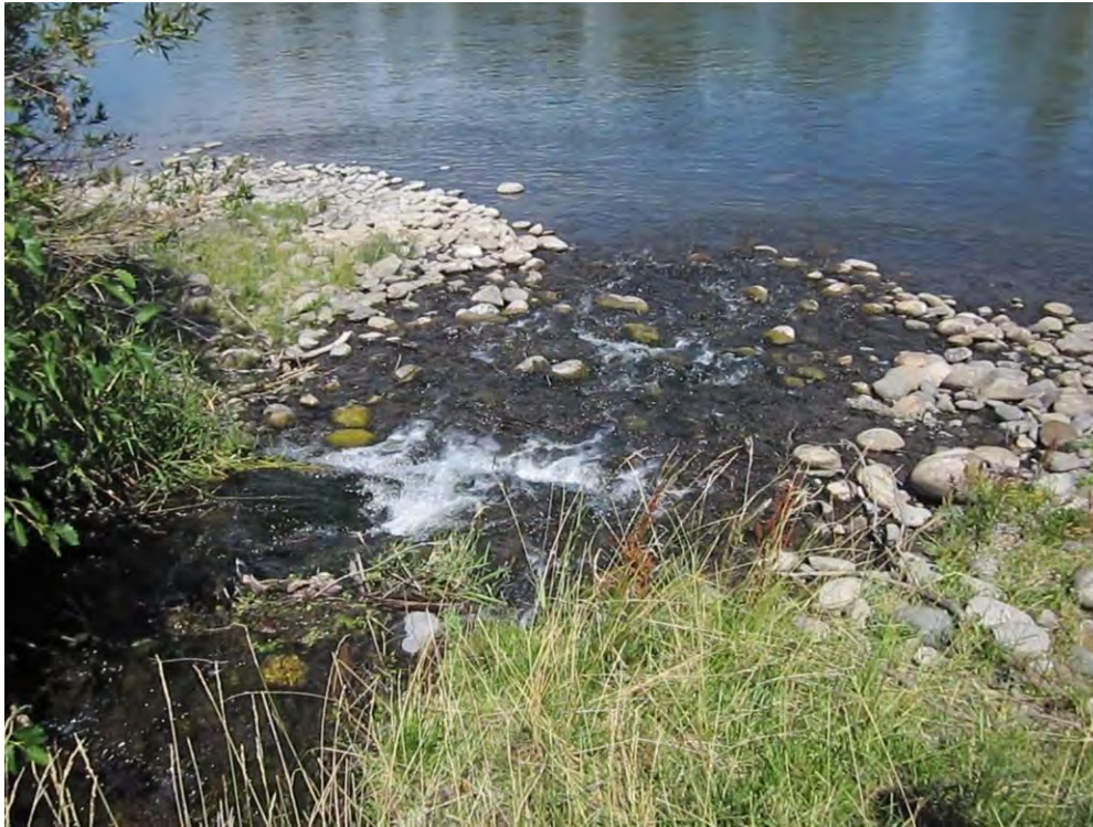
Figure 2-41. Confluence of Esp Spring Creek with the Yellowstone River, showing absence of constructed step-pools.
