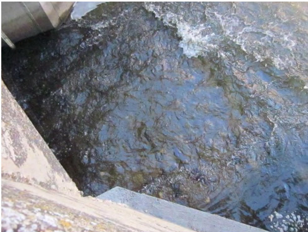
Figure 2-19. Outlet of box culvert on Clear Creek
