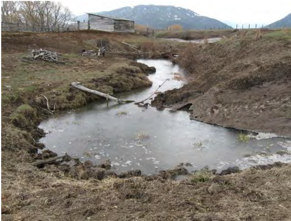
Figure 2-48. Pre-restoration view of Fleshman Creek.
