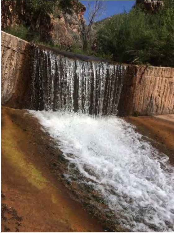
Figure 2-21. Splash pad of the Crooked Creek barrier.
