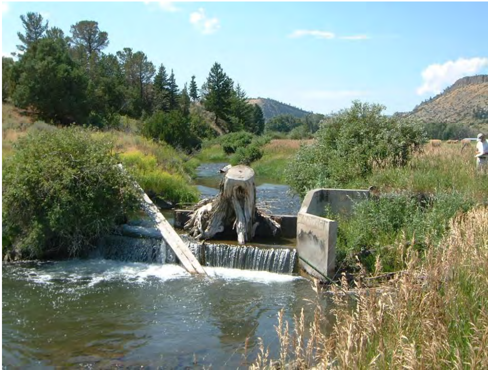
Figure 2-10. Irrigation diversion blocking fish passage on Brackett Creek (2003).
