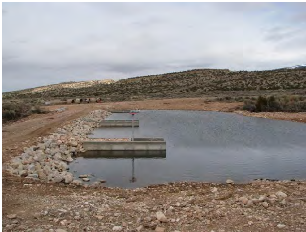
Figure 2-70. Storage pond and gated stand pipes soon after construction.
