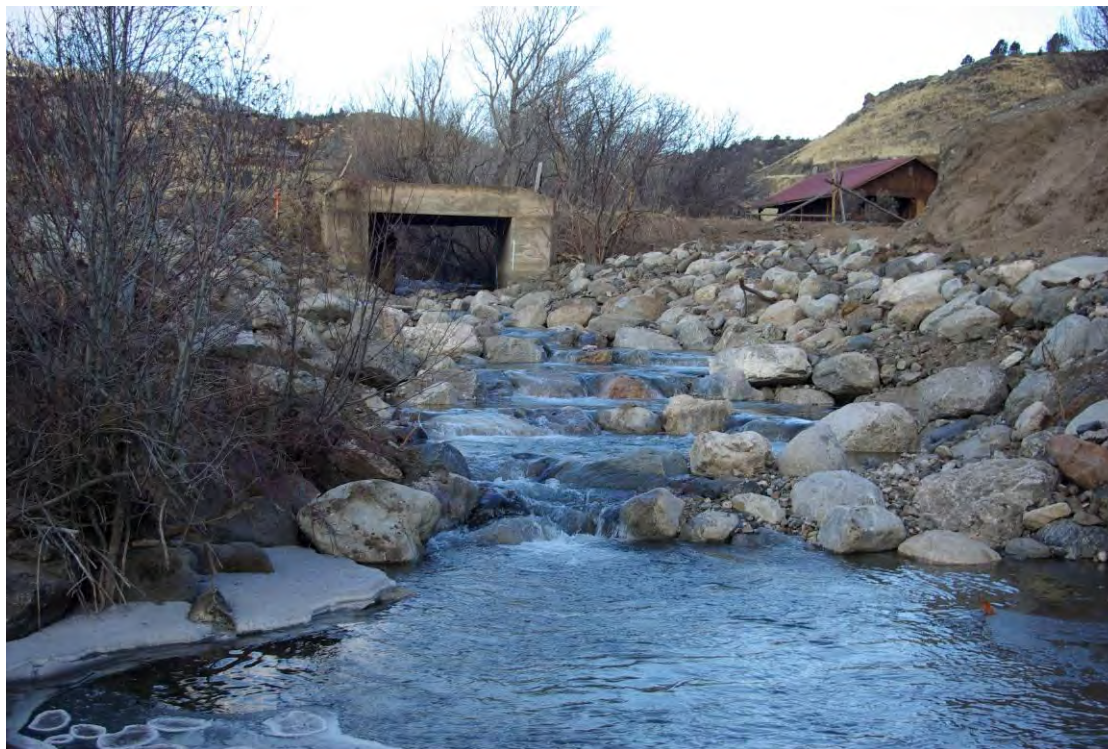
Figure 2-73. Newly constructed step-pool sequence.
