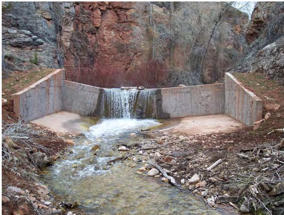
Figure 2-20. Newly constructed barrier on Crooked Creek, 2008.
