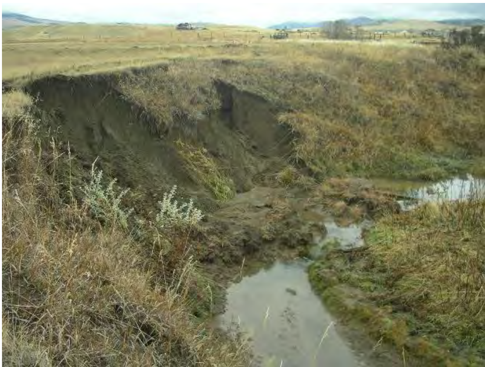
Figure 2-49. Example of an eroding terrace on Fleshman Creek within the project area.
