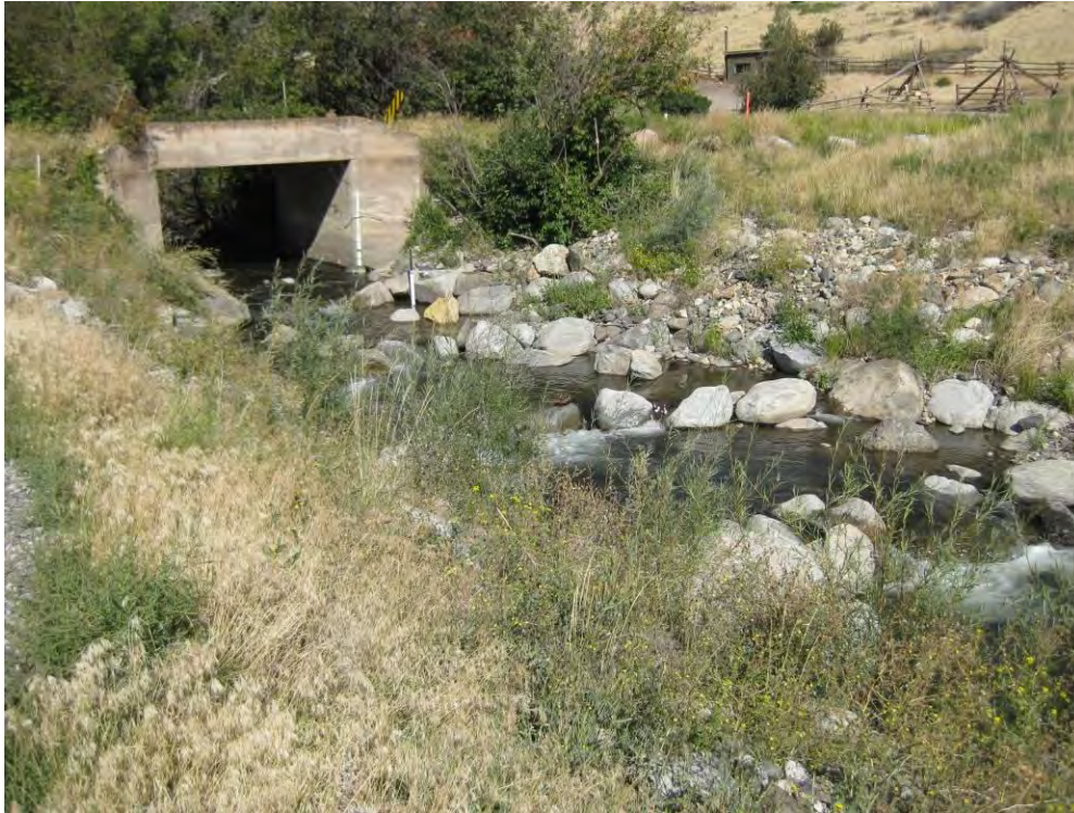
Figure 2-74. Step-pool sequence constructed to provide fish passage into Rock Creek.
