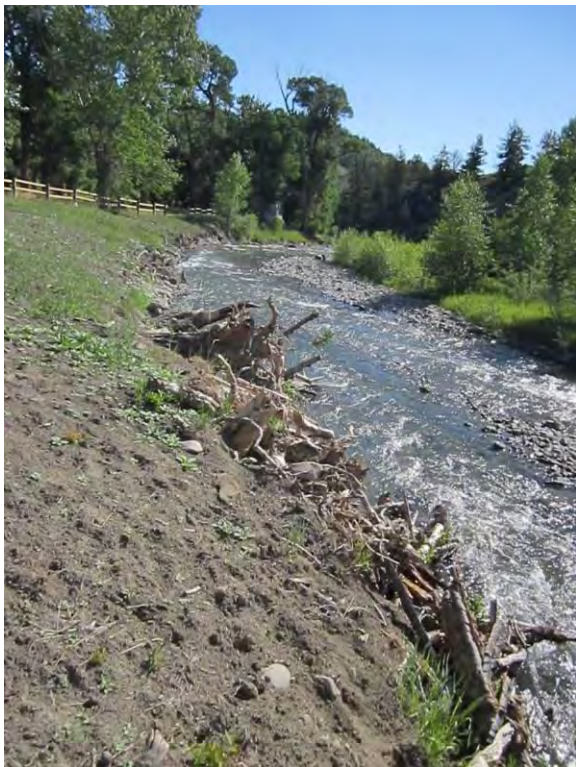
Photo 5. Root wad and log revetment installed in April 2016.
