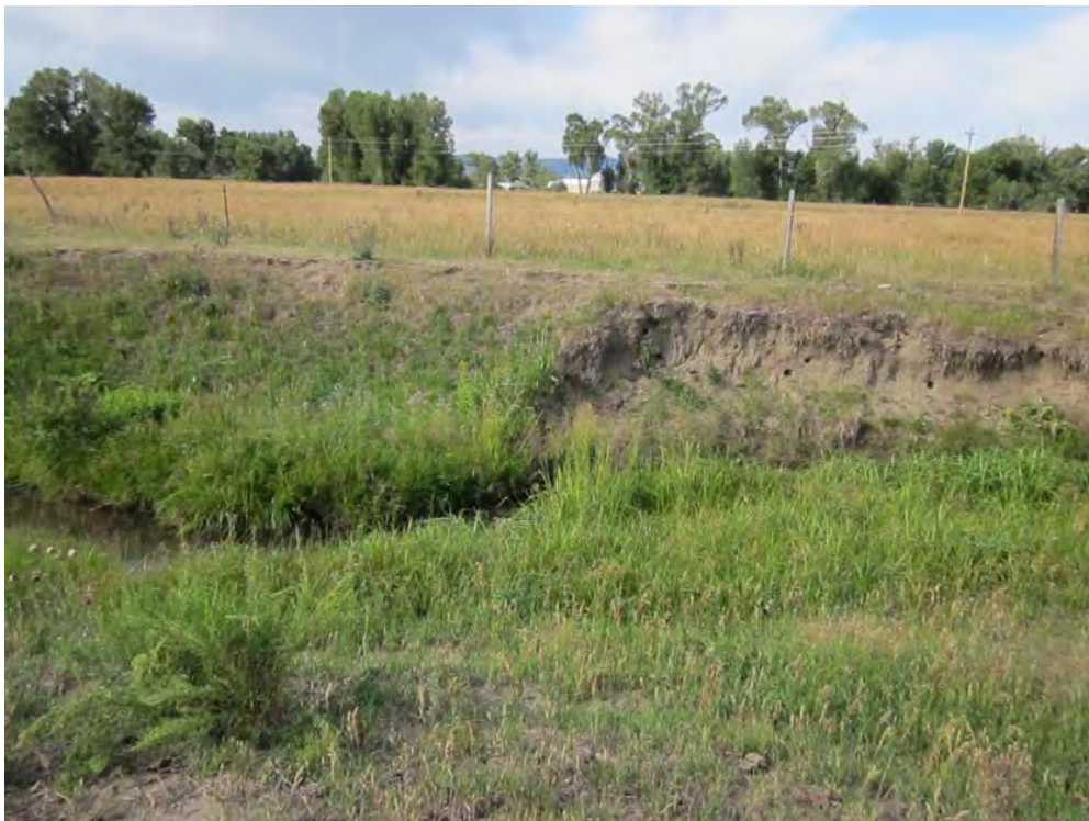
Photo 11: Evidence of 2011 flood demolishing part of the bank.
