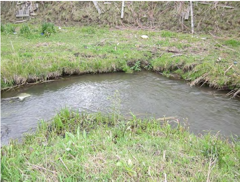
Photo 3: Some bank sloughing.
