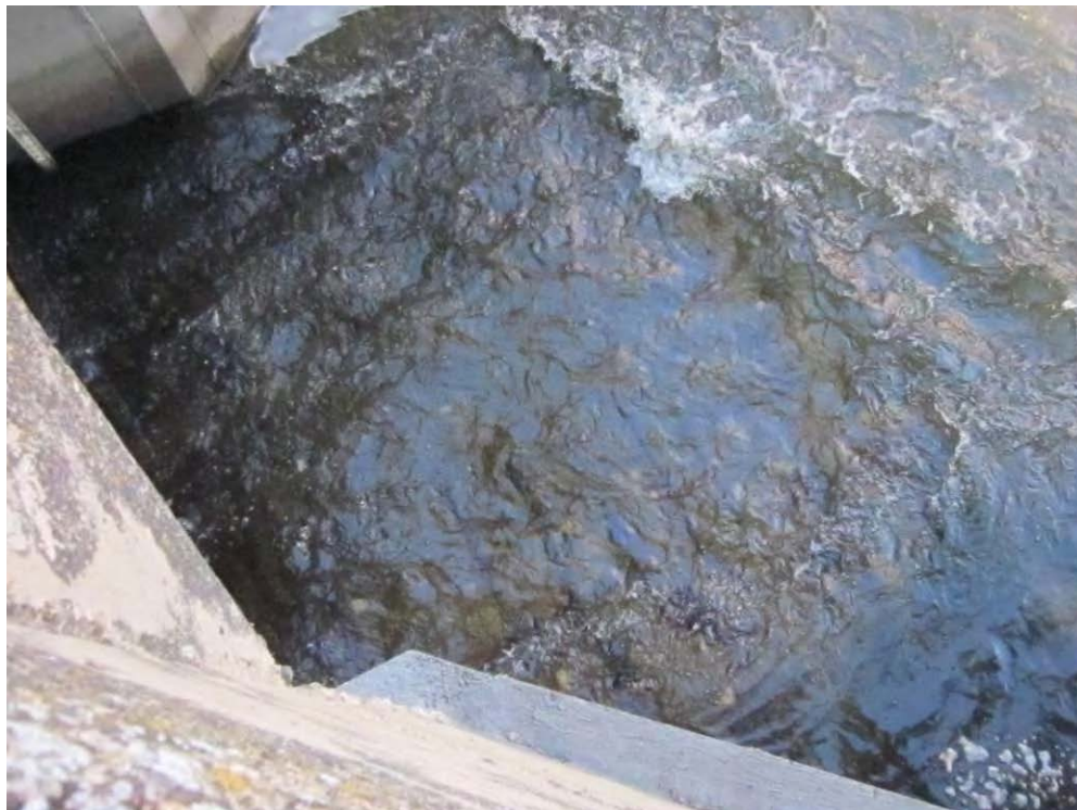
Photo 1. Bridge with pool up to bottom of culvert.
