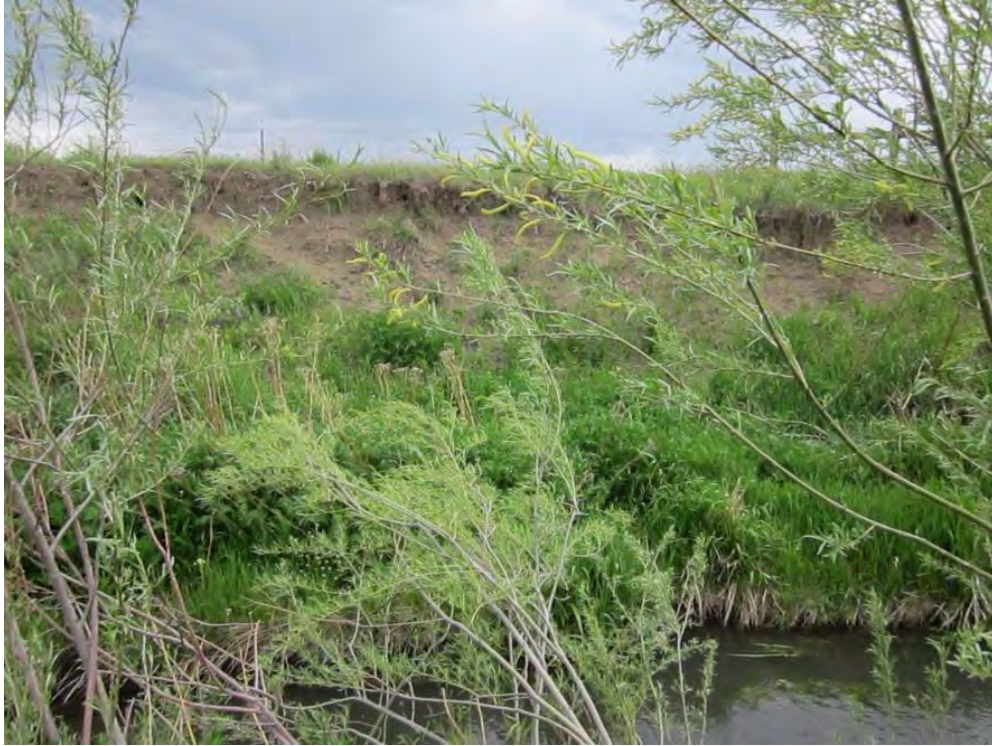
Photo 10: Floodplain bench still in working condition.
