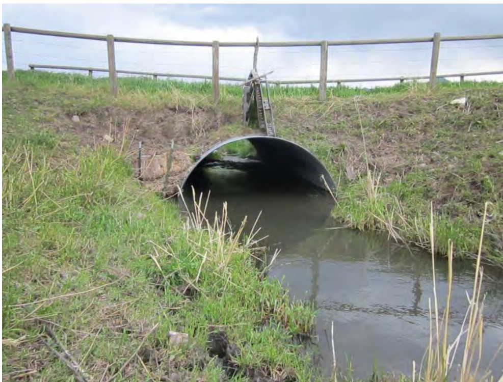
Photo 9: Second bottomless culvert.
