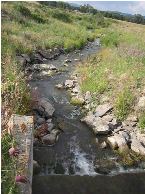
Photo 3: start of project. (head gate on Elk Creek)
