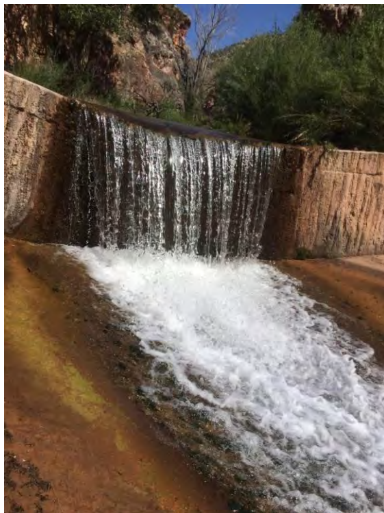
Photo 1. Splash pad in good condition, and not providing passage over structure
