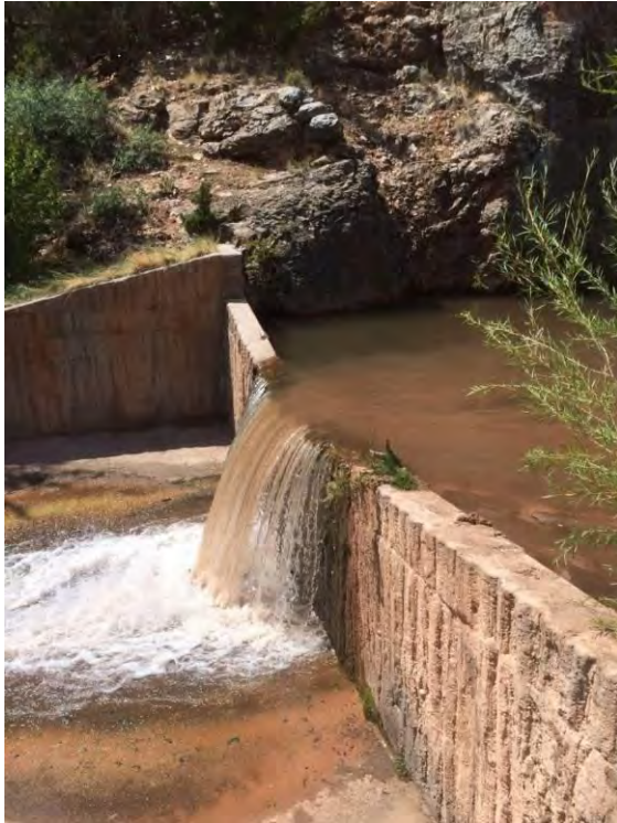
Photo 2. Accumulation of gravel behind wall of barrier forming a solid surface.
