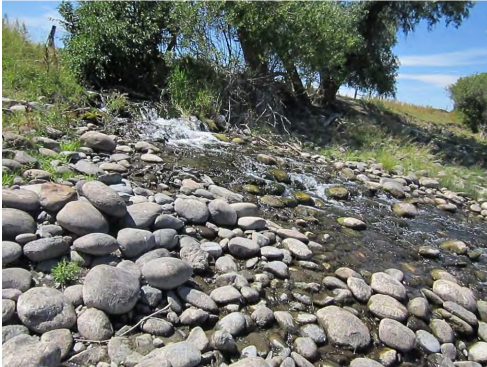
Photo 2: Start of project should have step-pools, but larger rocks have been displaced do to possible ice jams.
