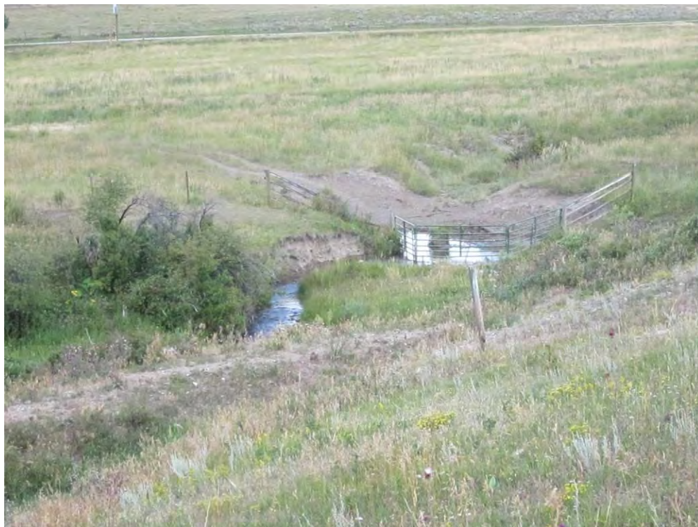
Photo 5: Emergency stock water.
