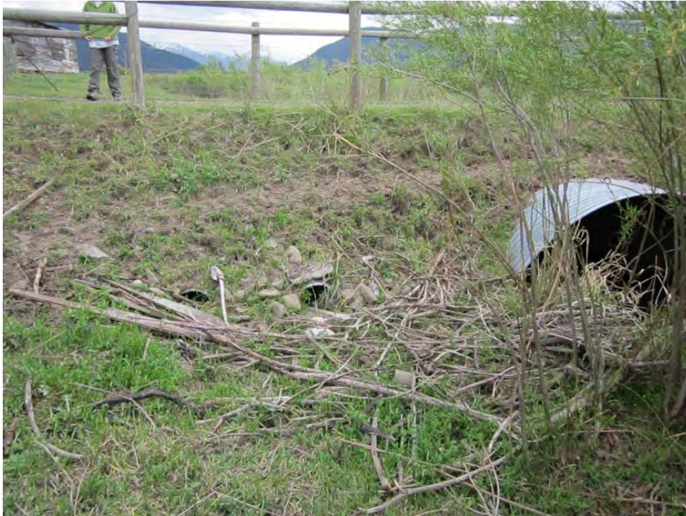
Photo 6: Bottomless culvert and overflow.
