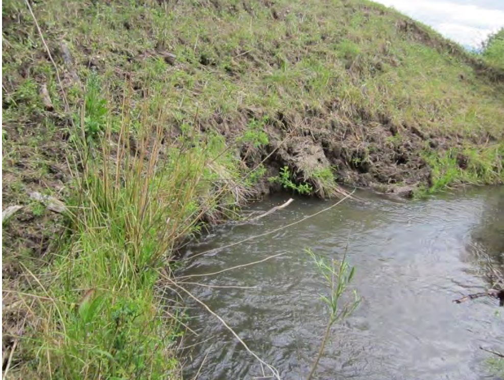
Photo 8: Cattle trail resulting in bank erosion.
