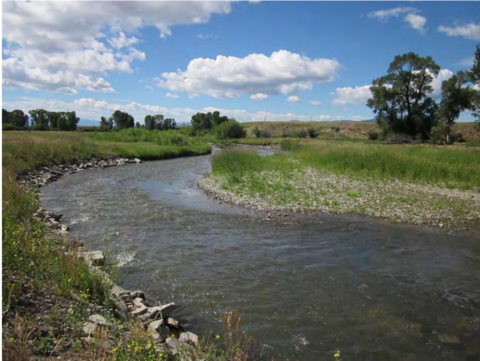
Photo 3. Rock armoring at toe of bank.
