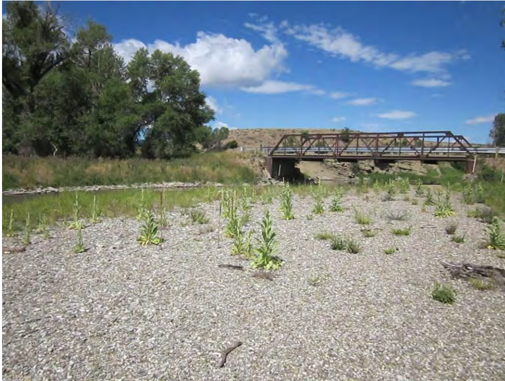
Photo 1. Point bar and bridge at start of project
