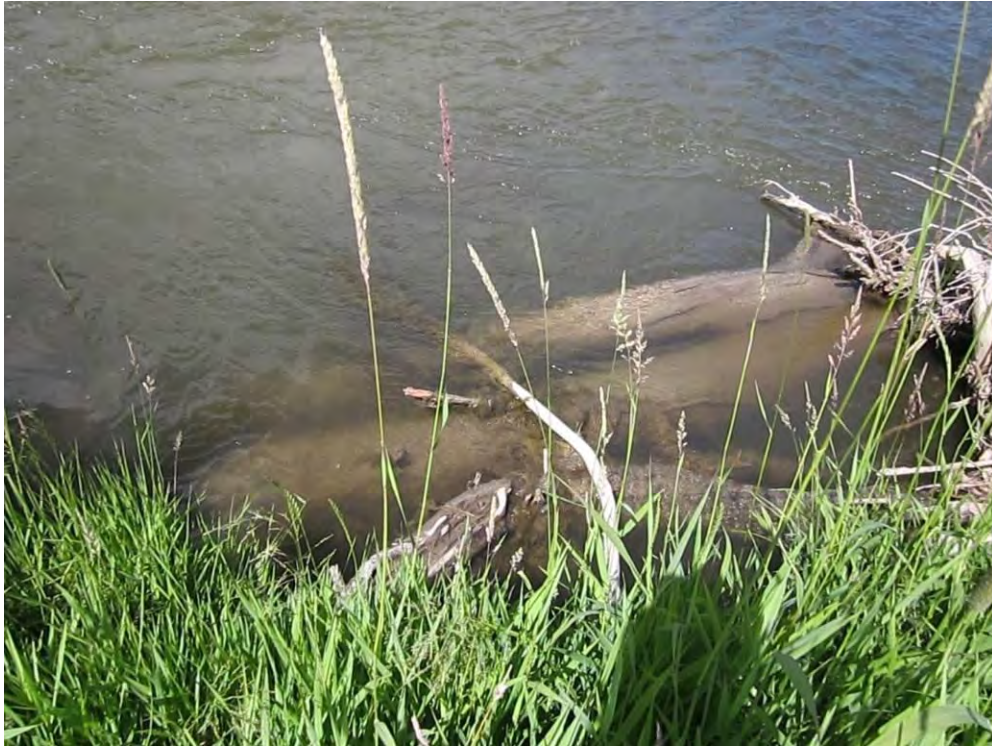
Photo 5. Root wad and tree revetment.
