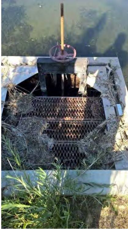
Photo 2. Evidence of regular cleaning of screen
