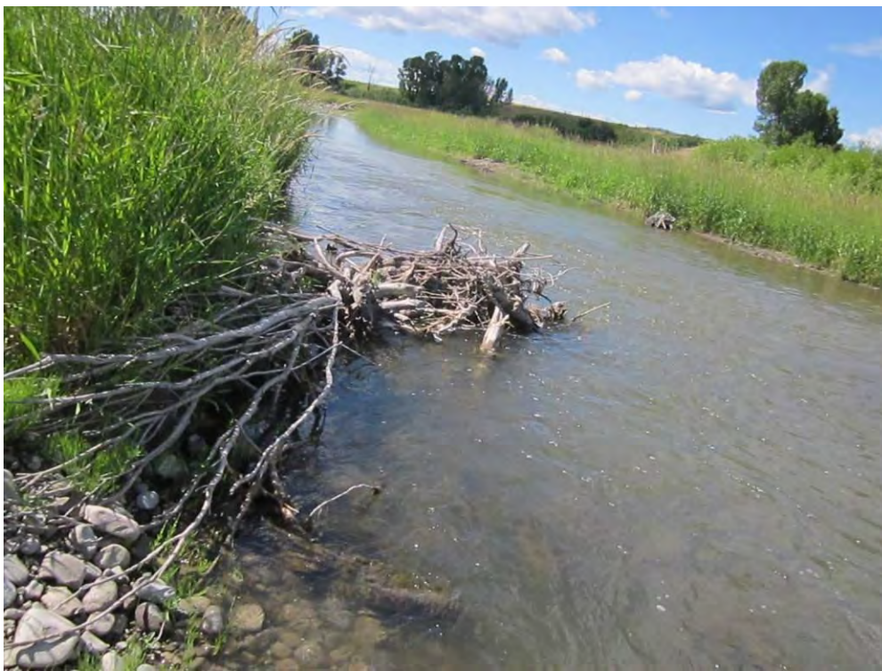
Photo 4. Root wad and tree revetment.
