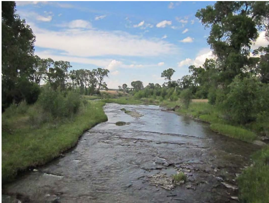
Photo 1: Bridge at start of project
