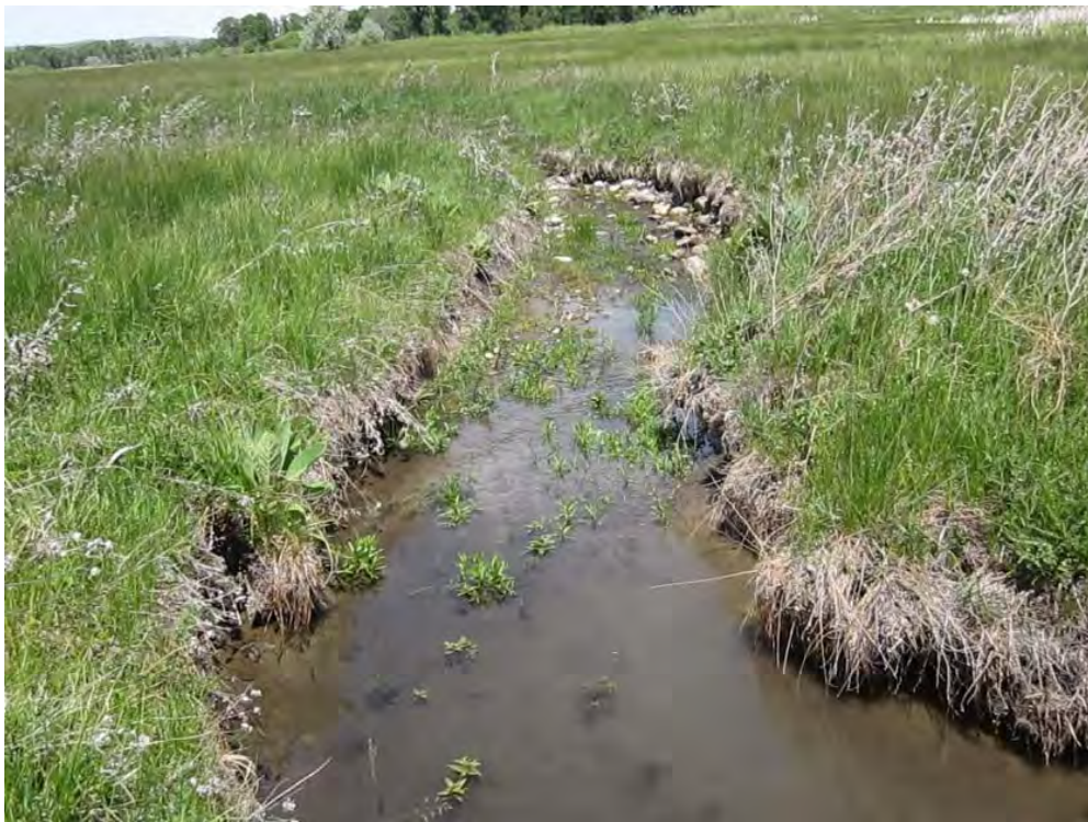
Photo 7: Pool full of sediment, higher grade=exposed gravel.
