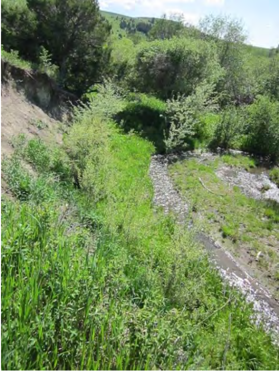
Photo 7: Floodplain bench working
