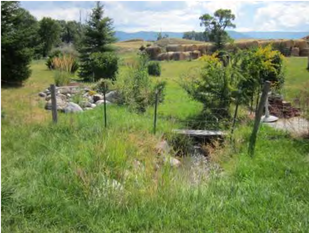
Figure 8. Current view of the relocated spring creek.
