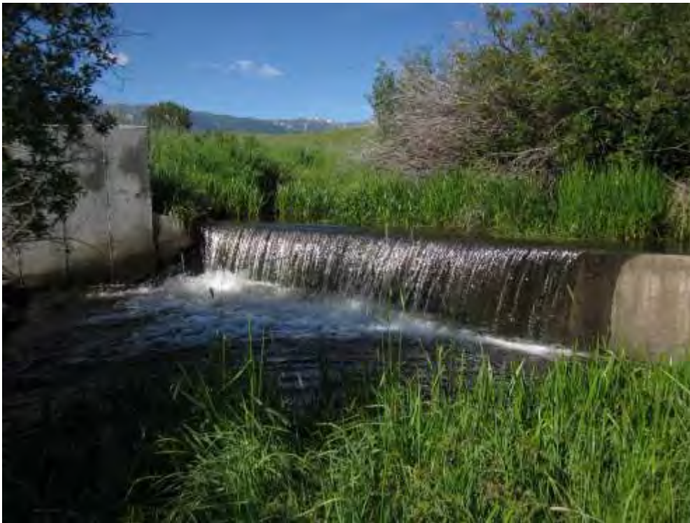
Figure 103. The Thiel Creek fish barrier.
