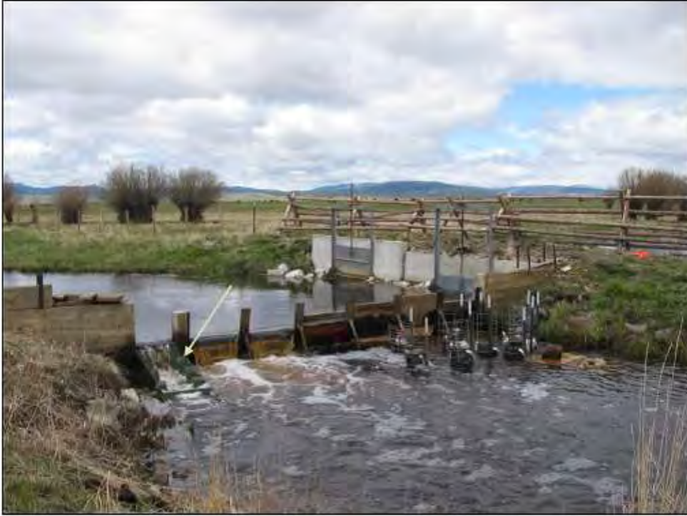
Figure 2. Example of pin and plank irrigation diversion equipped with Denil fish ladder and screw gate typical of those being installed in Big Hole River watershed to protect Arctic grayling, and the stated conceptual approach for the diversion on Cottonwood Creek.
