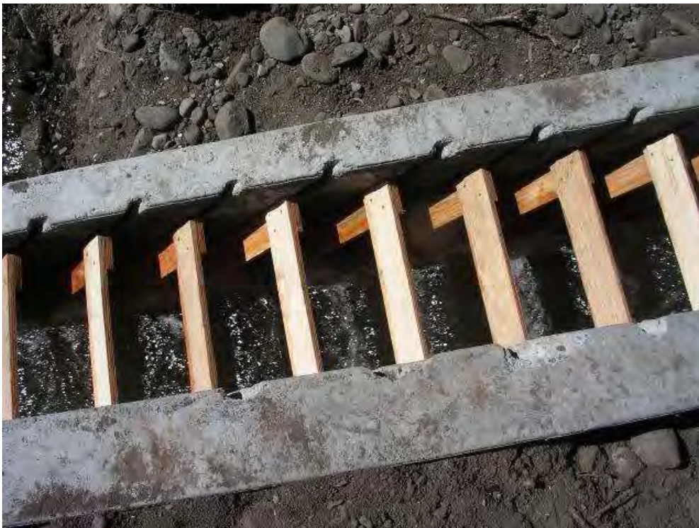
Figure 90. Wooden baffles in the South Fork Fridley Creek fish ladder.
