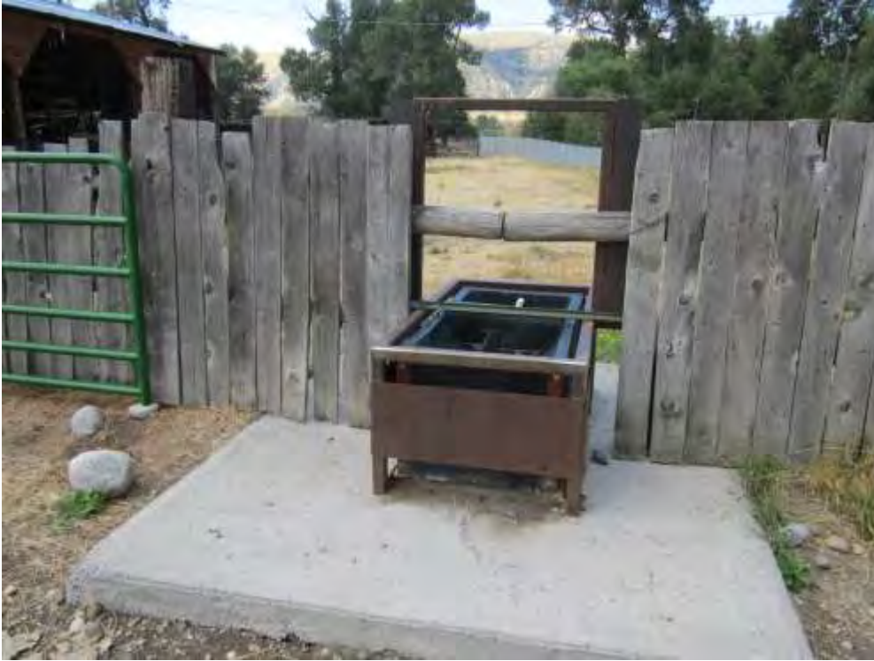
Figure 9. Example of an off-stream water source for corrals installed as part of this project.
