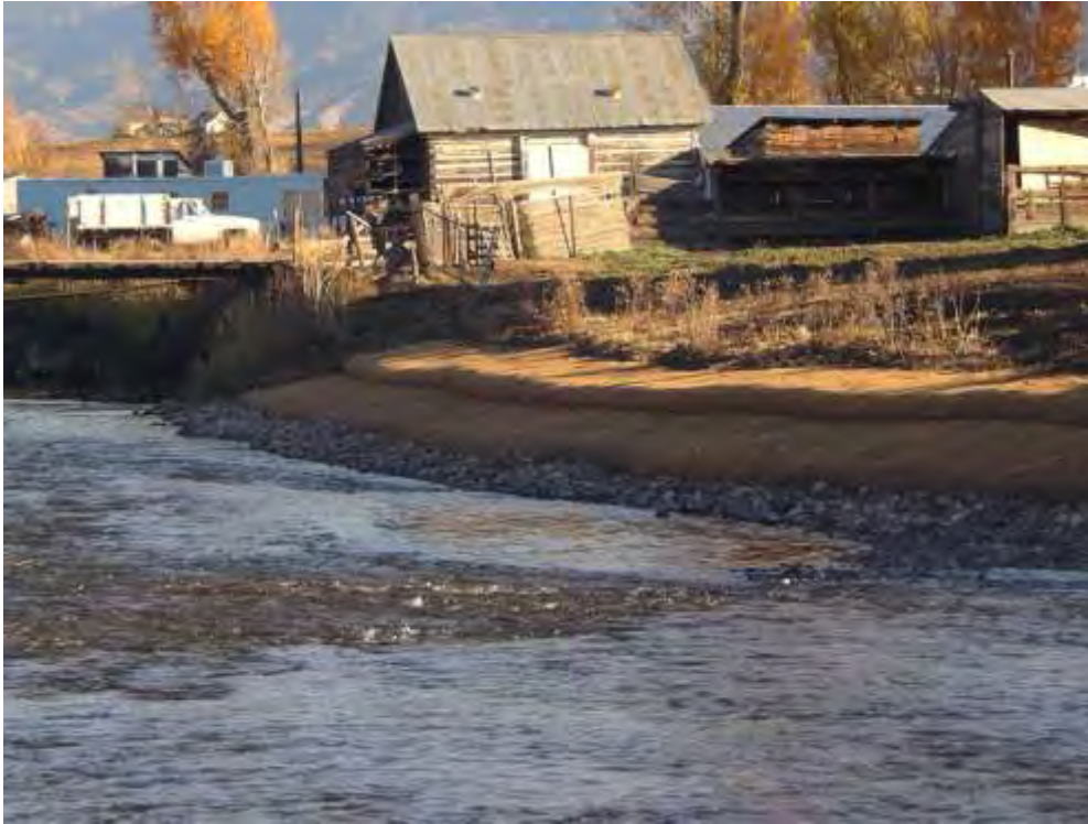
Figure 14. Example of fabric-encapsulated soil lifts on bank 2.
