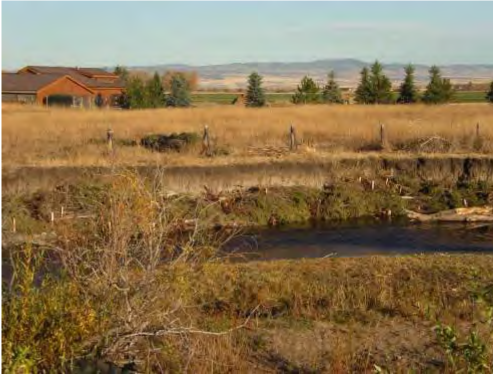
Figure 15. Juniper revetments cabled into bank 3.
