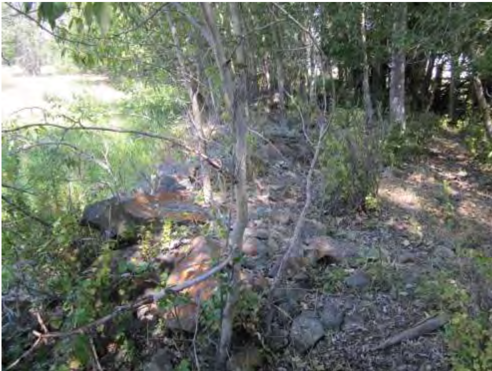
Figure 83. Old riprap that was no longer near the channel.
