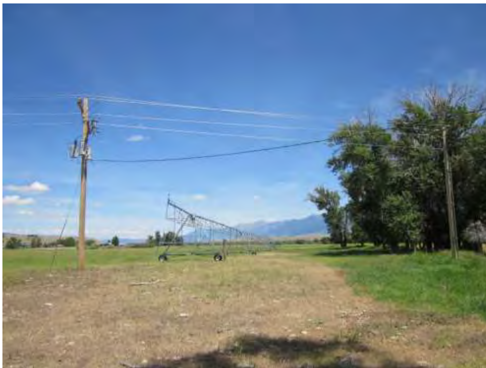
Figure 33. Center pivot installed as a water savings measure for North Fork Fridley Creek.
