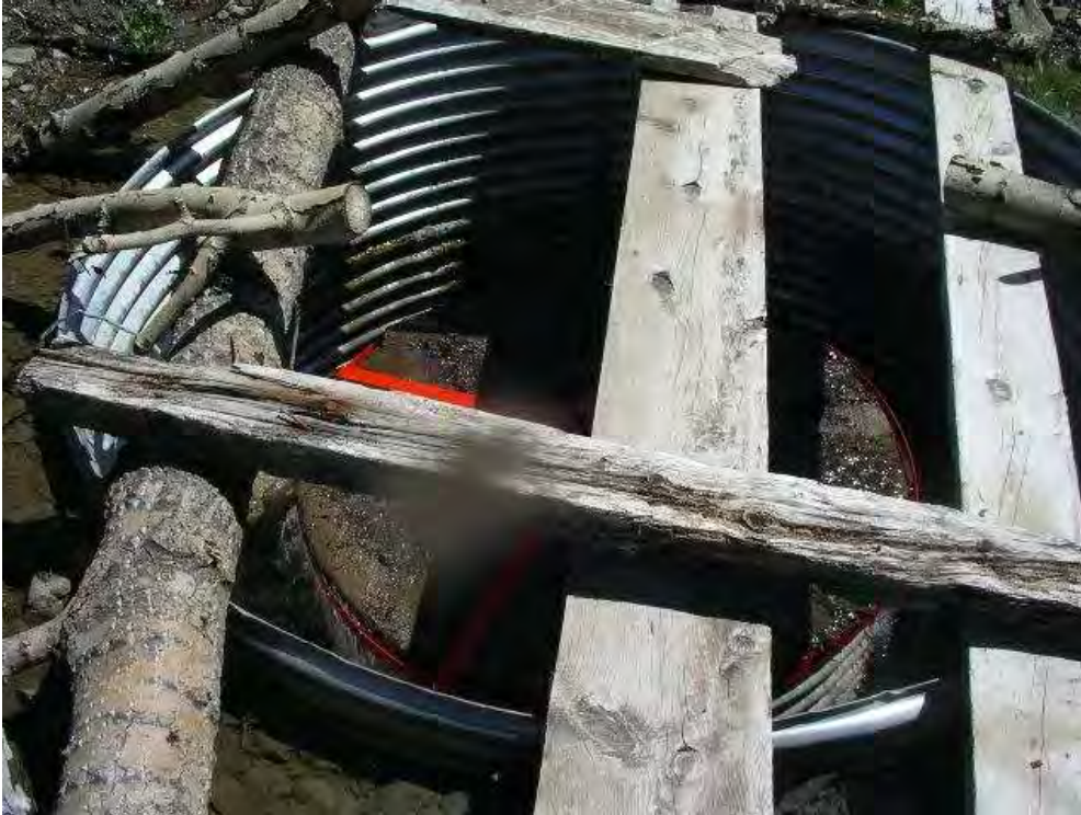
Figure 50. Turbulent fountain screen when not in use.
