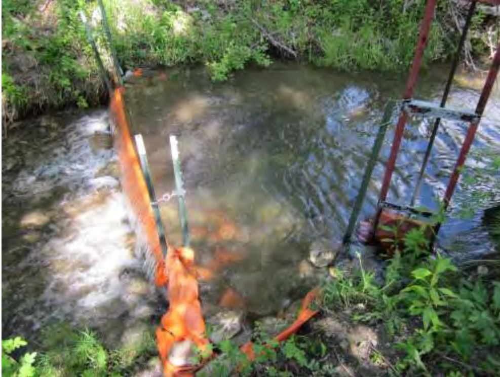
Figure 53. Check boards impounding flows to deliver water to the head gate.
