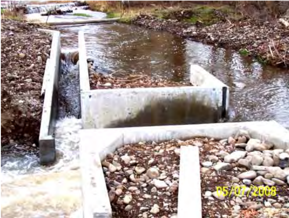
Figure 89. Newly constructed fish ladder on South Fork Fridley Creek
