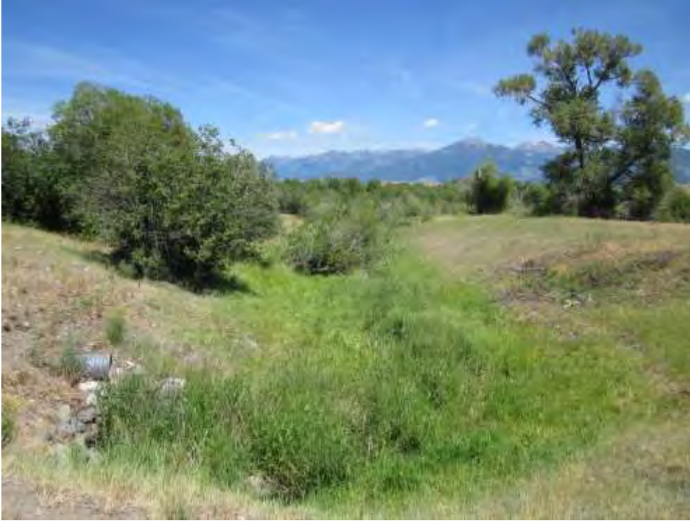
Figure 31. North Fork Fridley Creek emerging from downstream end of siphon under Park Branch Canal.
