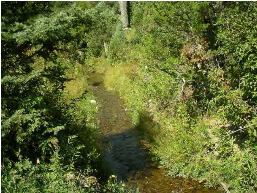
Figure 4. Water leaking into ditch on Cottonwood Creek when check boards were blocking flow.
