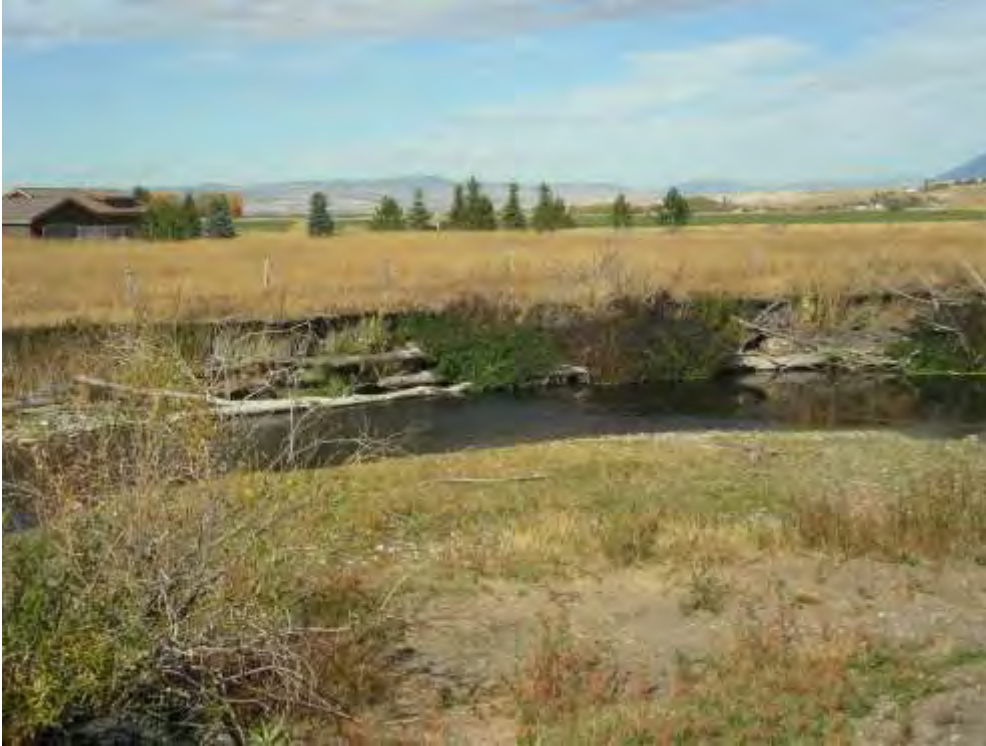
Figure 12. Bank 3 on the East Gallatin River, showing cabled in cottonwoods that were part of an earlier bank stabilization effort.
