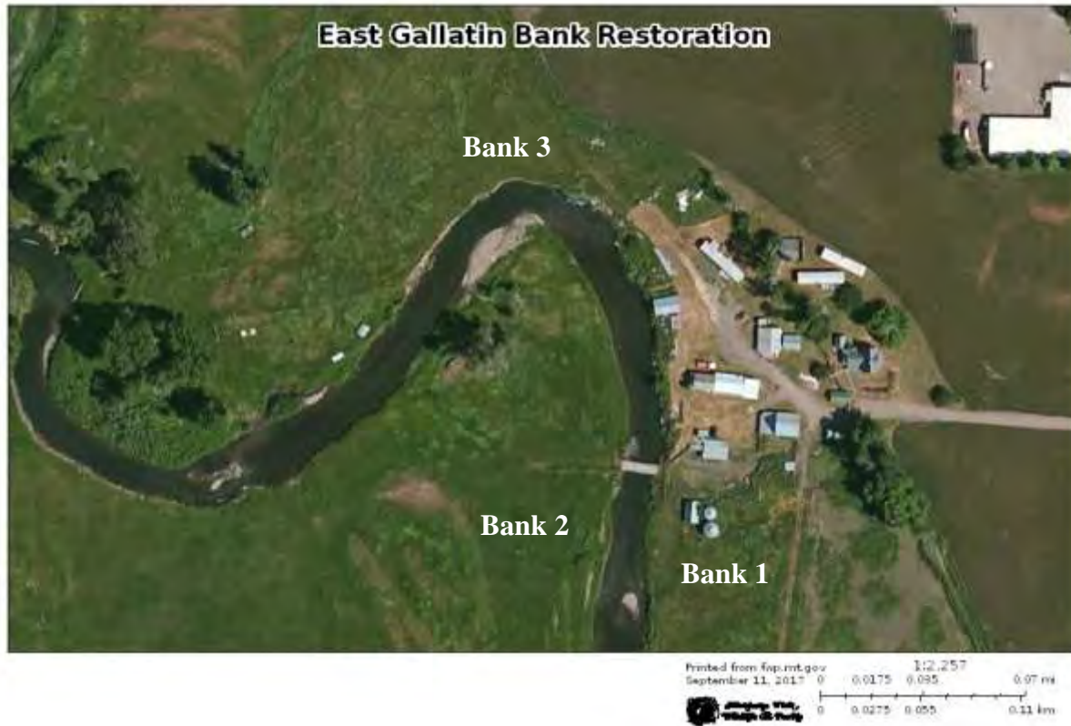
Figure 16. Aerial view of the project area showing locations of the three treated banks.
