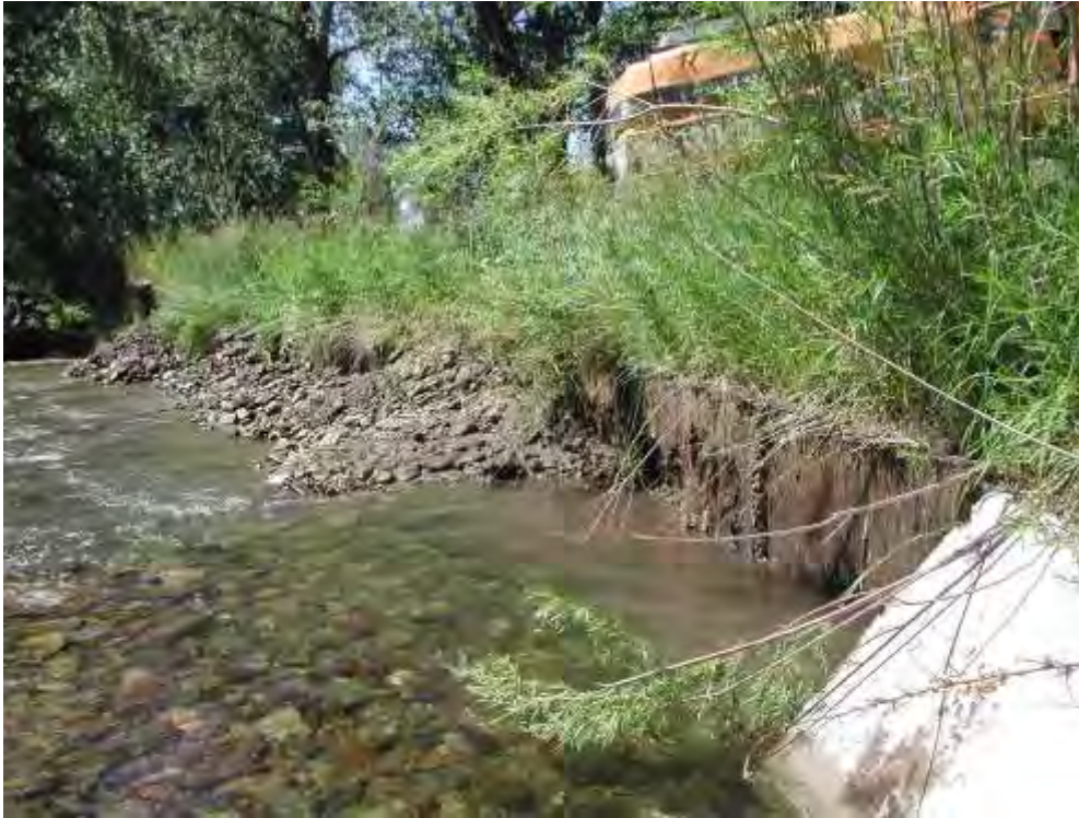
Figure 63. Removal of Concrete block and installation of a rock toe.
