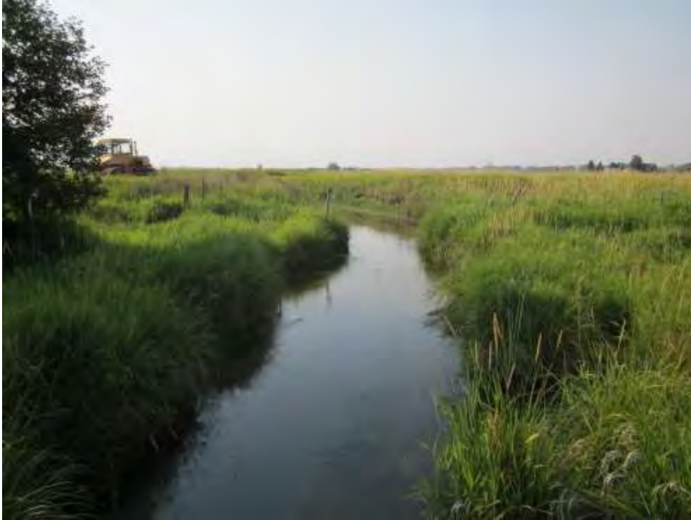
Figure 97. Overly wide channel on restored portion of South Fork Ross Creek.
