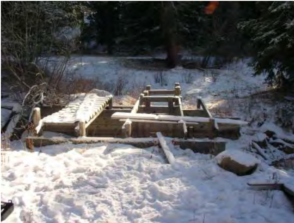
Figure 45. Pin and plank irrigation diversion on North Fork Horse Creek.
