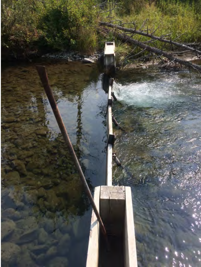
Cottonwood Creek Diversion Replacement (004-08)
