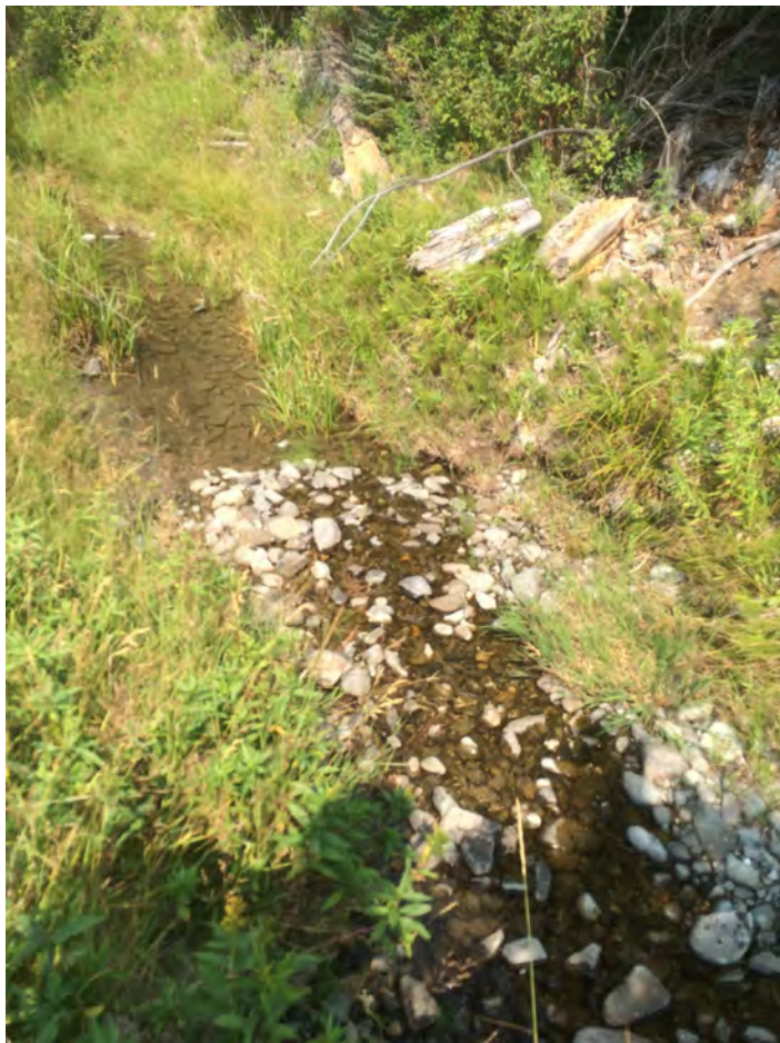
Cottonwood Creek Diversion Replacement (004-08)
