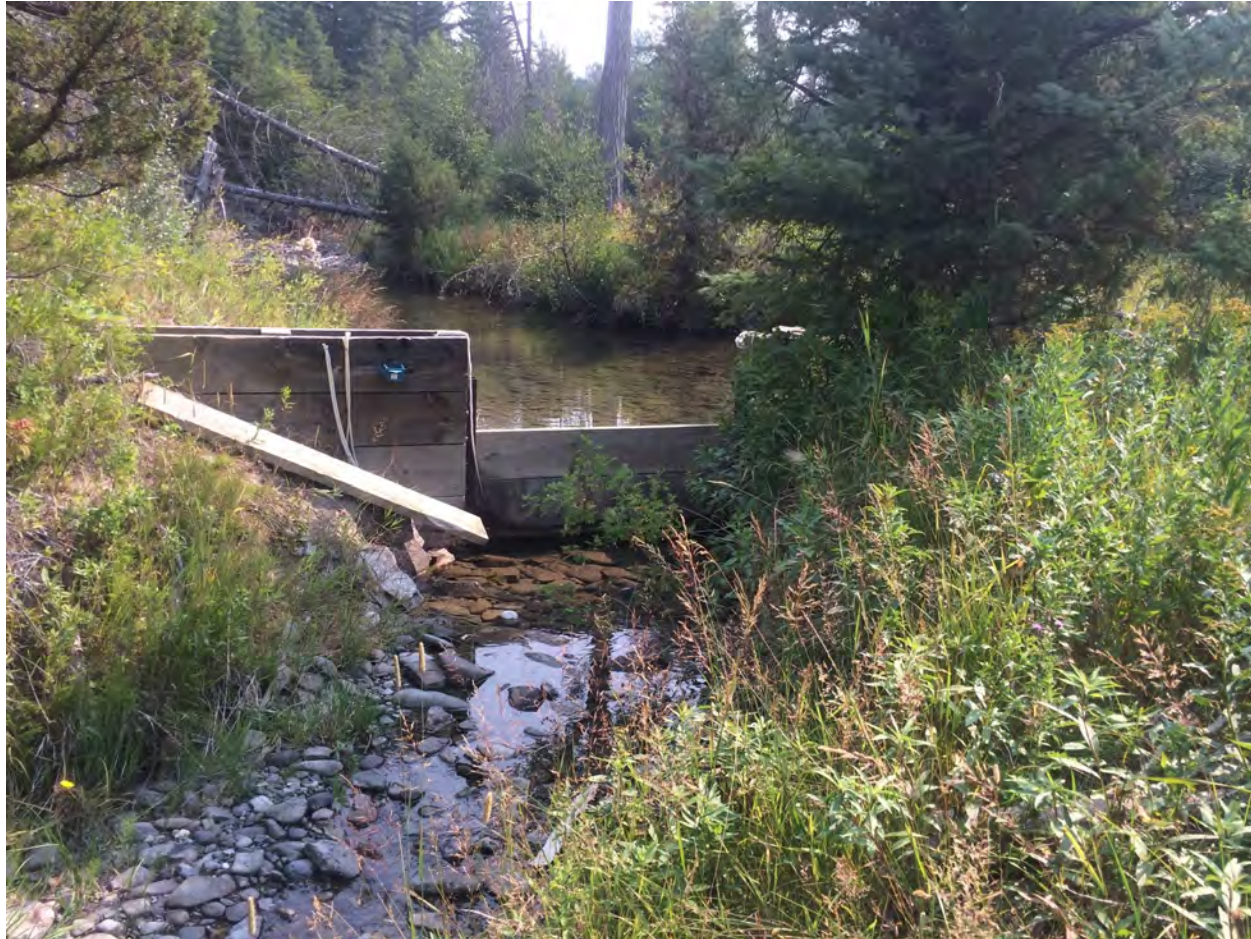
Cottonwood Creek Diversion Replacement (004-08)
