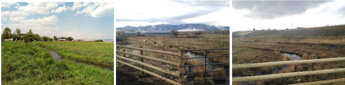
Before After (fencing; note, different project viewpoints)
