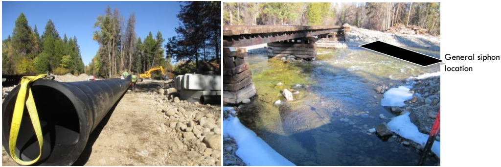
During (siphon pipe)
