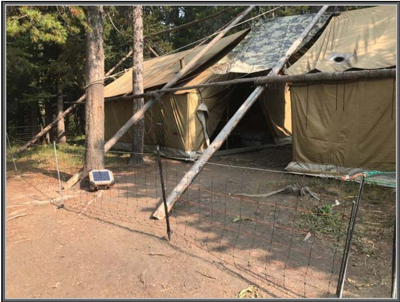
A temporary electric fence with a 12-volt battery and solar panel charger was installed around an outfitter camp in the Bob Marshall Wilderness Area.
