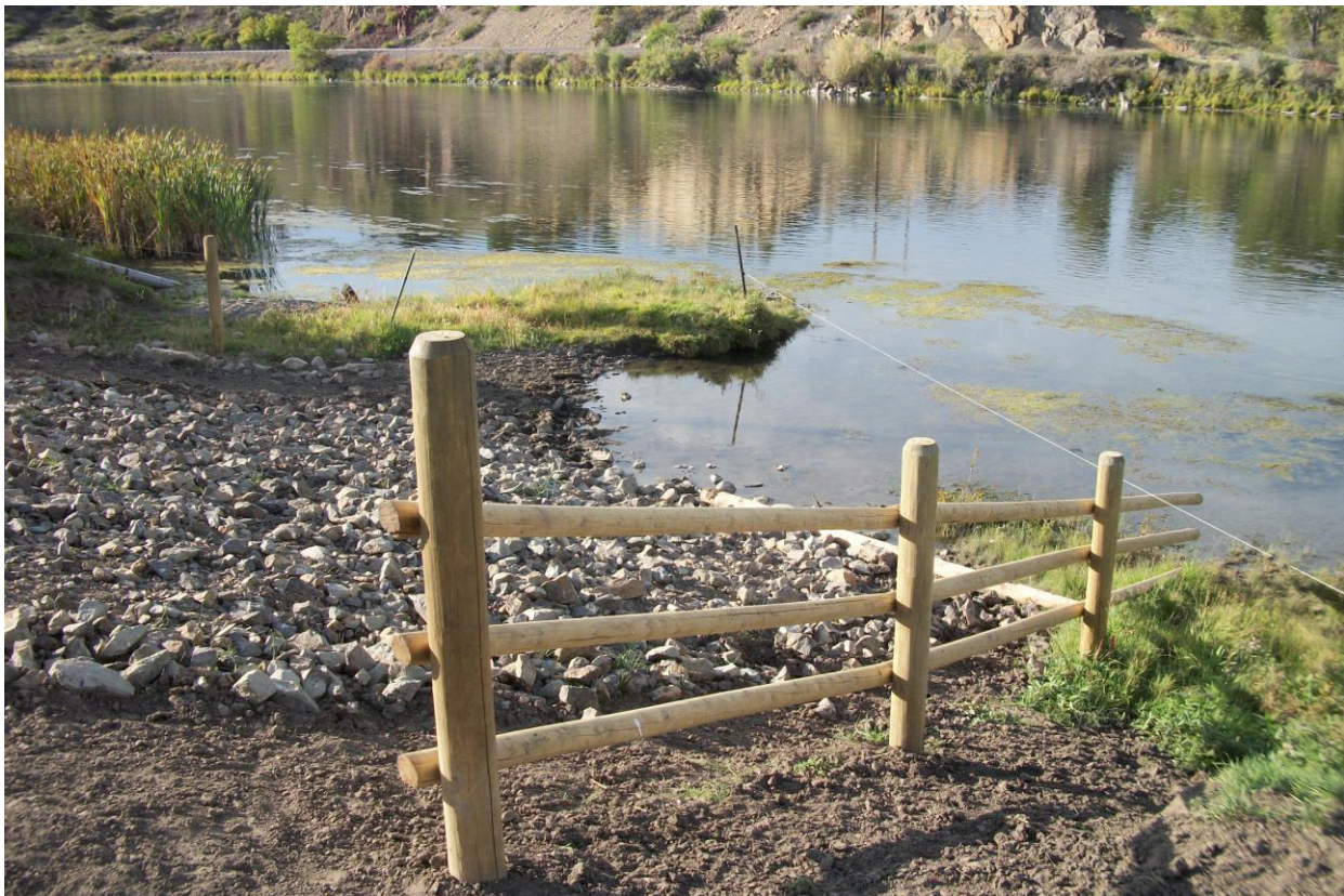
South Pivot water gap – upper. Note; set posts are in place in background. Rails will be installed following irrigation intake cleanout. Sterling Ranch, Missouri River, Craig Montana.
