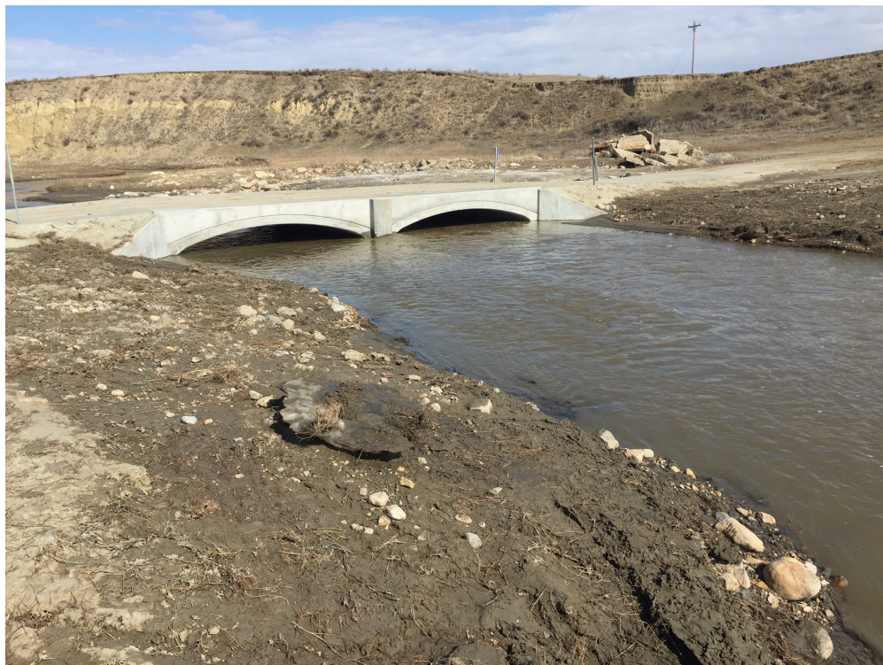
Photograph 2. Nickwall crossing after the two box culverts were installed.
